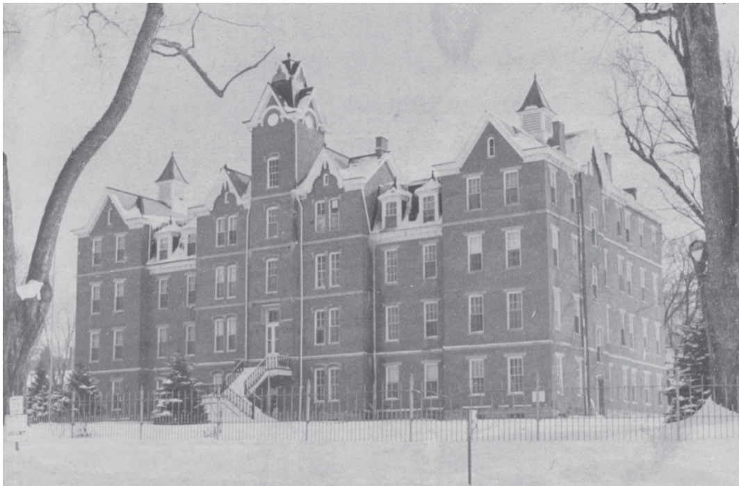
Figure 7. Knox County Infirmary c. 1880, displaying tripartite design, ample ventilation, large windows, and pleasing architectural style. (Courtesy of the Knox County Historical Society Museum.)
