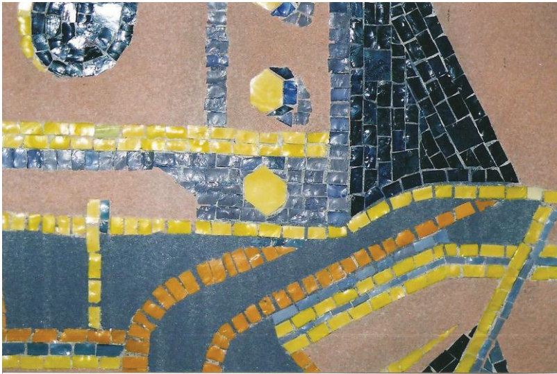
Figure 22 Picture showing that murals are a combination of mosaic and cement. Museum Center at Cincinnati Union Terminal
