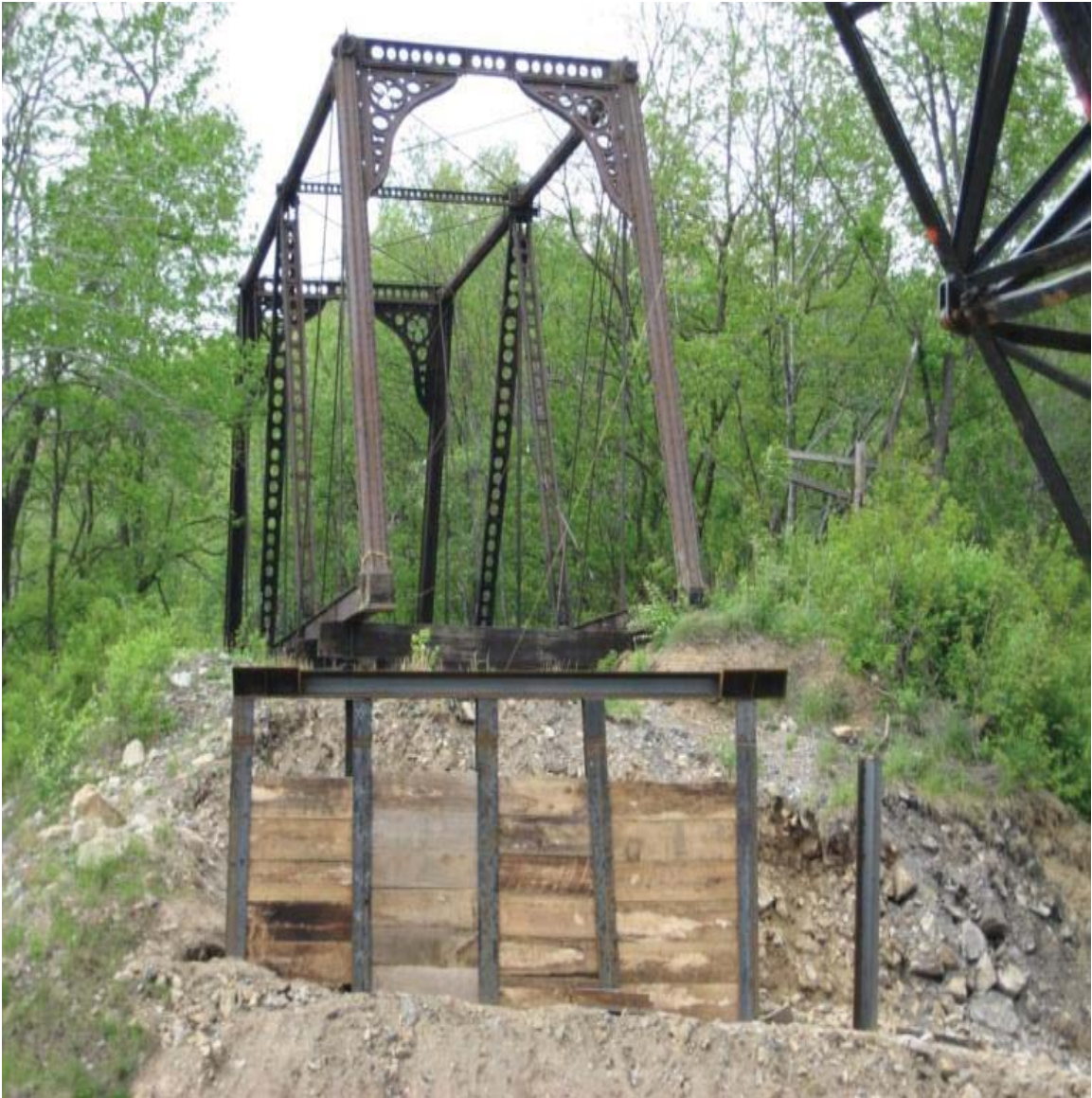
Figure 5-1: Relocating the Bollman Bridge to the Allegheny Highlands in 2007. Courtesy of Linda McKenna Boxx, Allegheny Trail Alliance
