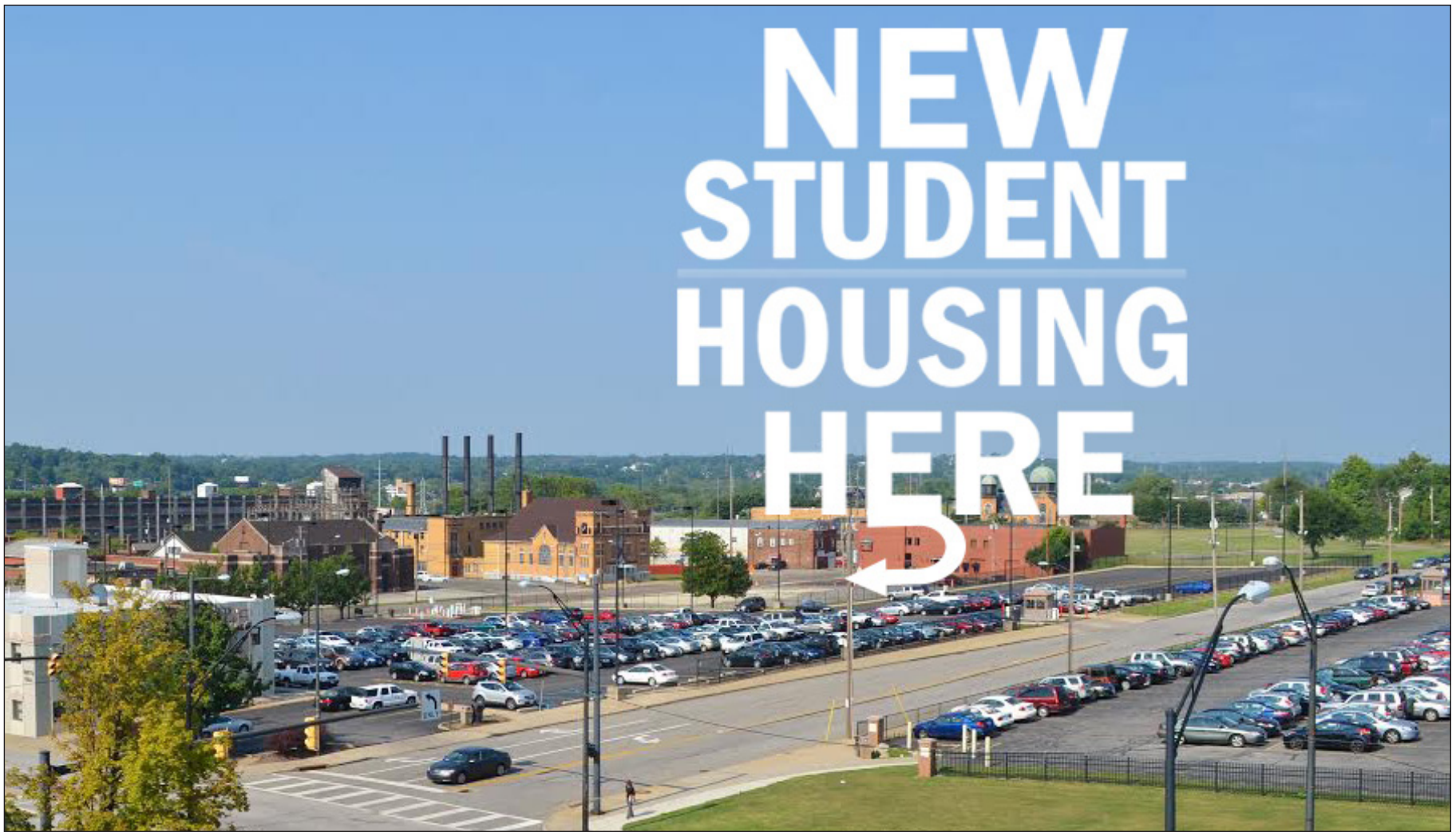
A new student housing complex will occupy the lot behind Smith Hall between Lincoln and Rayen Avenues.
