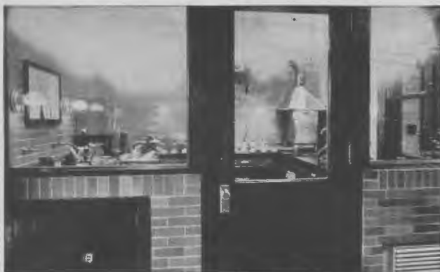
STEAM-WASHED PLATING ROOM where bacteriological analyses are made with every precaution to prevent contamination. All air taken into this glassed-in room is filtered. At frequent intervals, jets of live steam are employed to wash the air free of dust.
