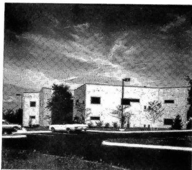
Ohtown Professional Building
