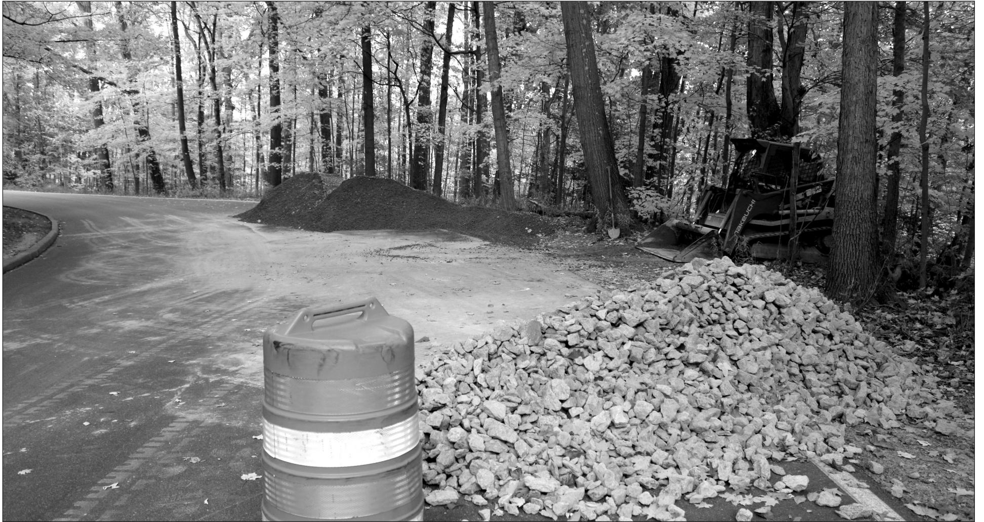
Trails will receive restorations and improvements for hikers.
