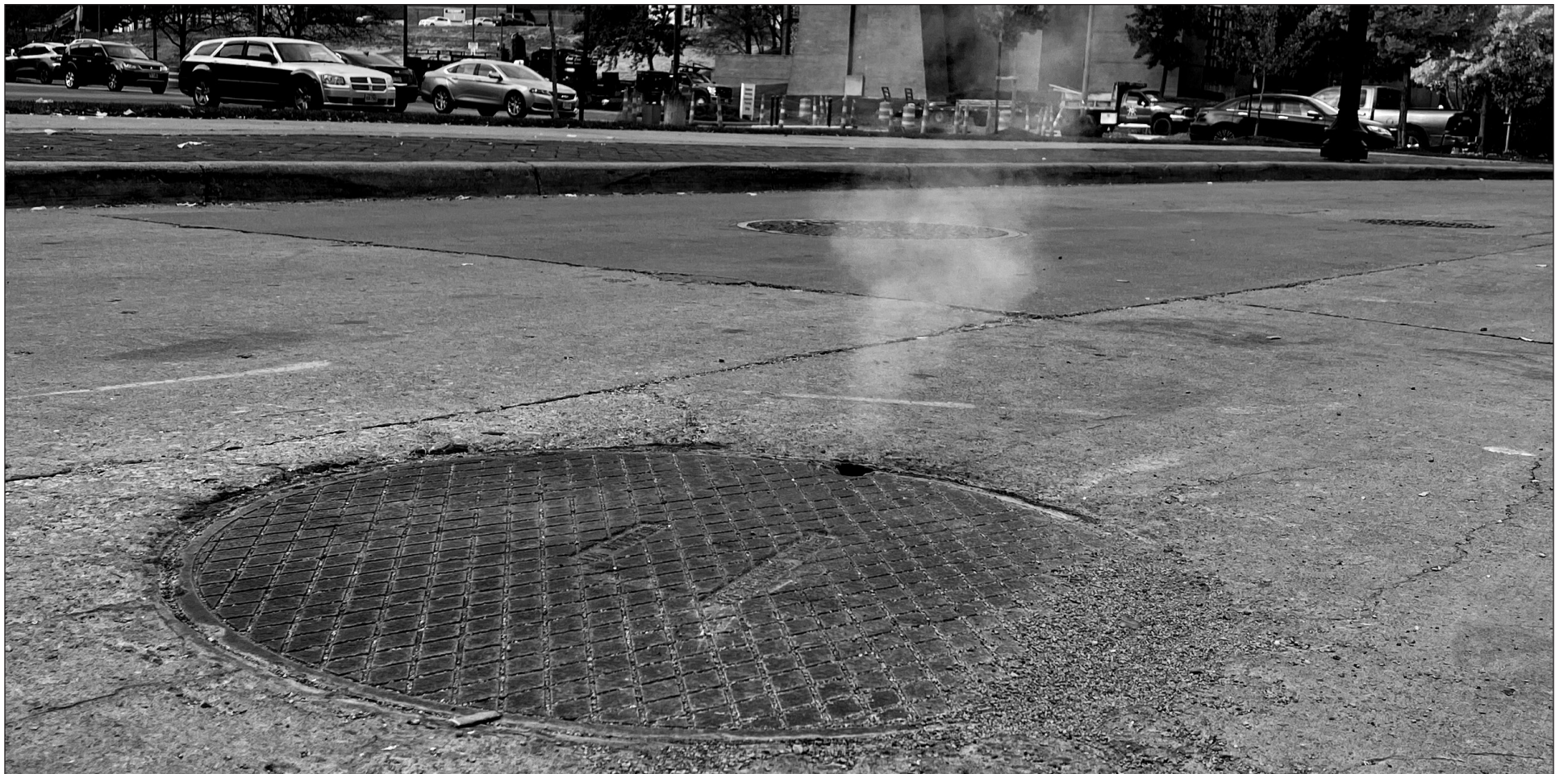
Steaming manhole in downtown Youngstown.
