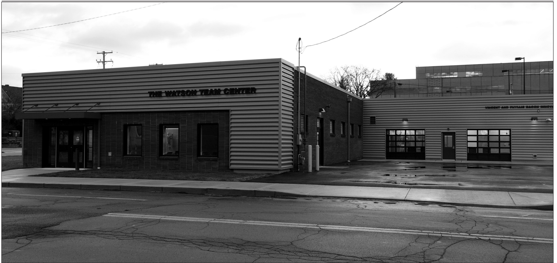
The Watson Team Center has been constructed in place of an old flower wholesaler.
