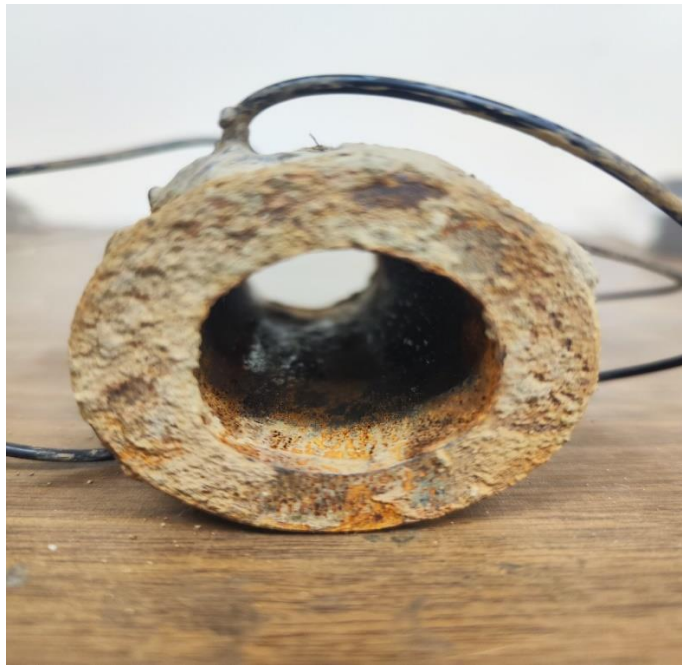
Figure 4.33. shows internal corrosion of metal buried under wet dirt.
