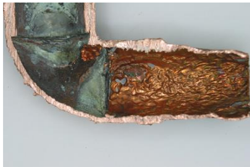
Figure 1.6. Erosion Corrosion on Inner Surface of an Elbow Pipe [110].
