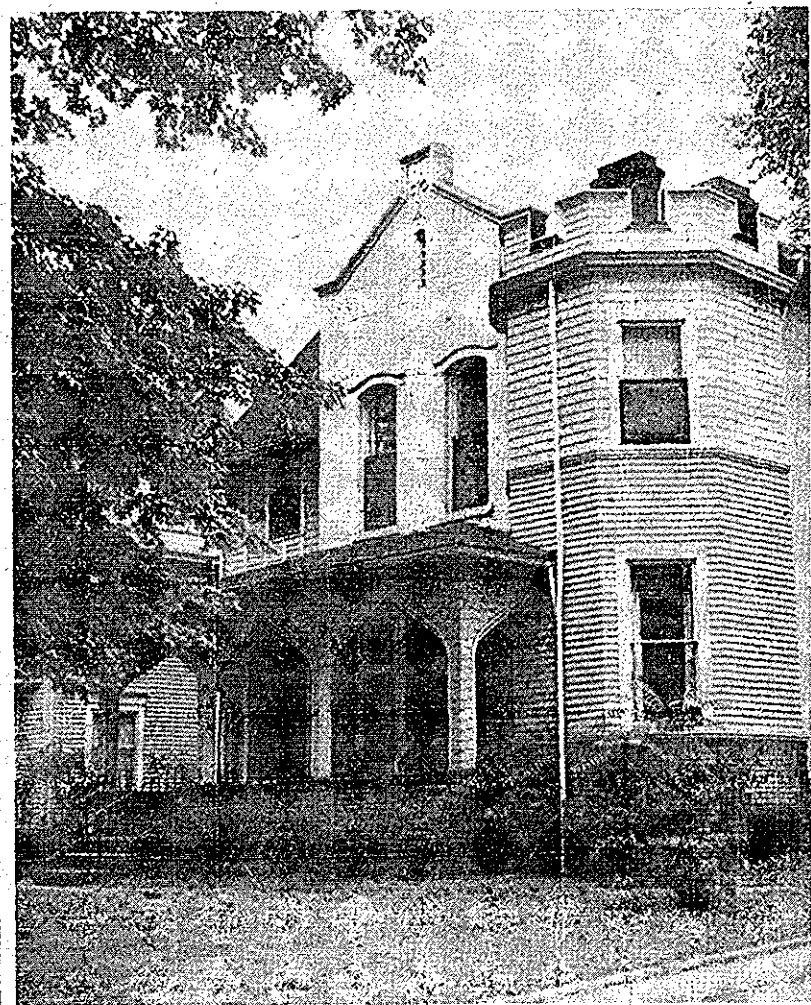
THETA CHI HOUSE: Pictured above is the new fraternity house, recently purchased by Theta Chi Fraternity. The house is located at 742 Bryson Street. (Photo by Paul Jagnow)
