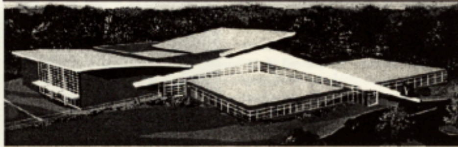
Davis YMCA/Wellness Center in Boardman
