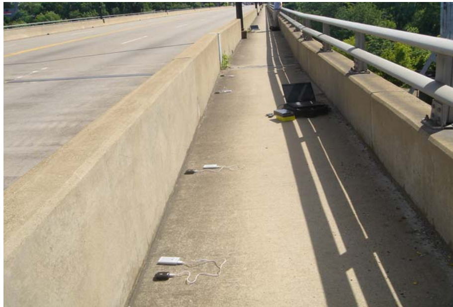
Fig. 4.3 Wireless sensor network deployed on bridge
