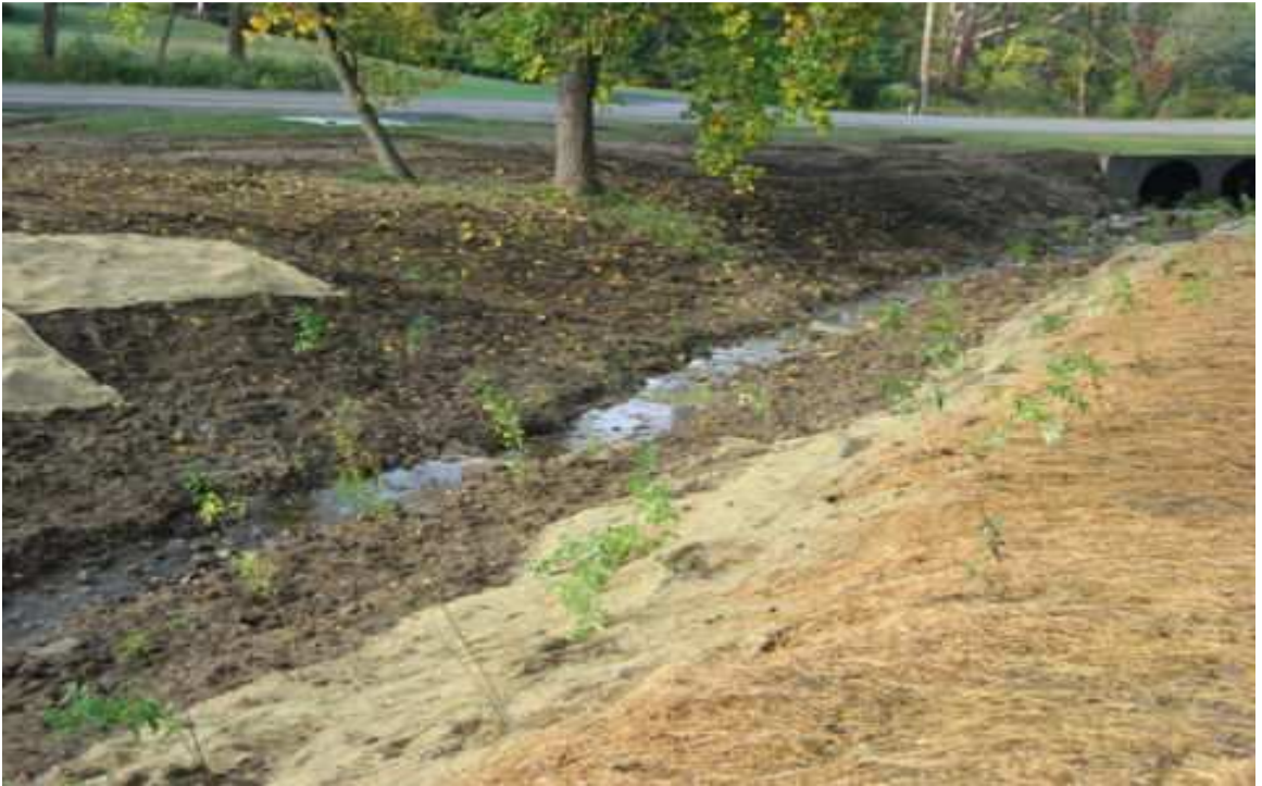
Figure 2.14 Planting riparian vegetation for Austintown Park project (WPI 2008).
