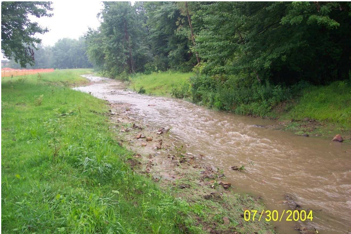
Figure 4.9 Meander pattern in restored reach of Indian Run (WPI 2004).
