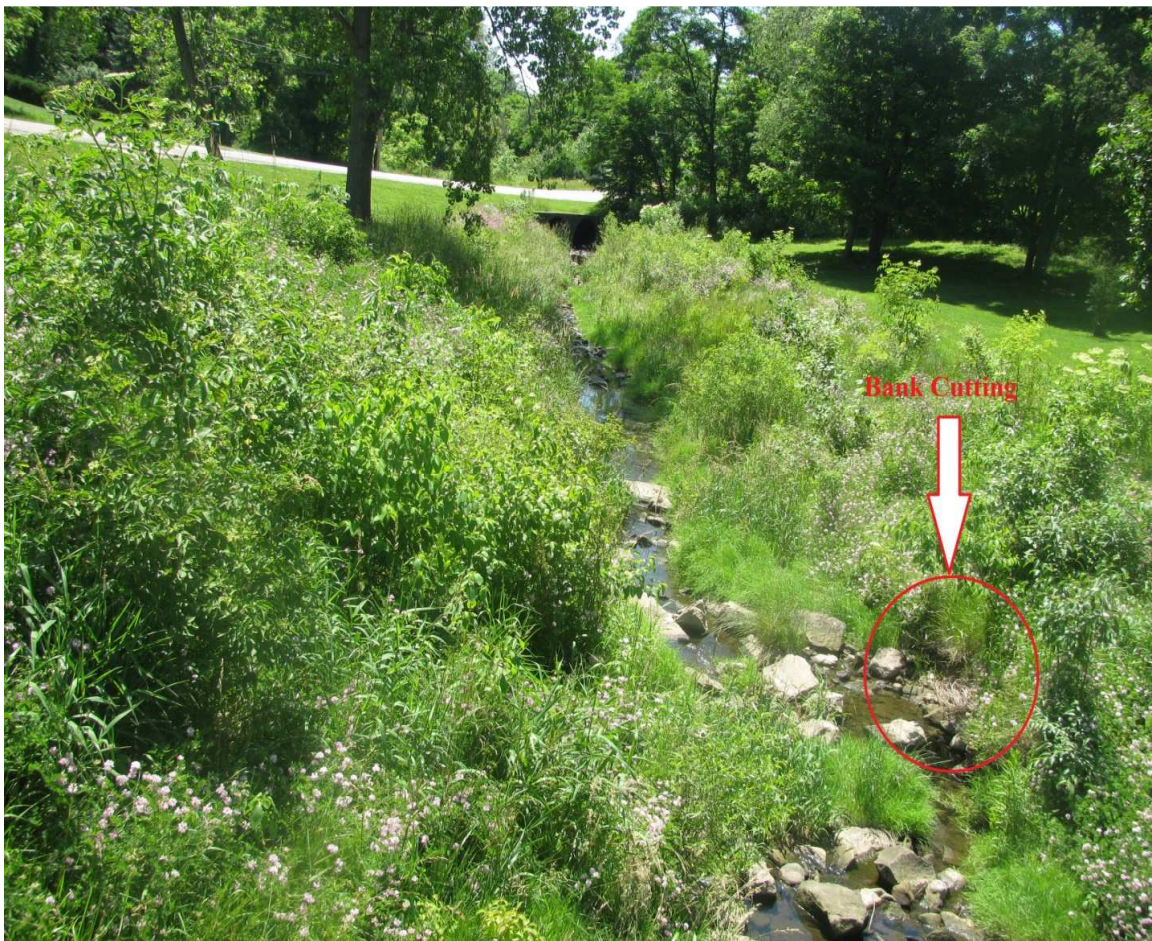
Figure 4.11 Bank cutting at Austintown Park site (June 2010).
