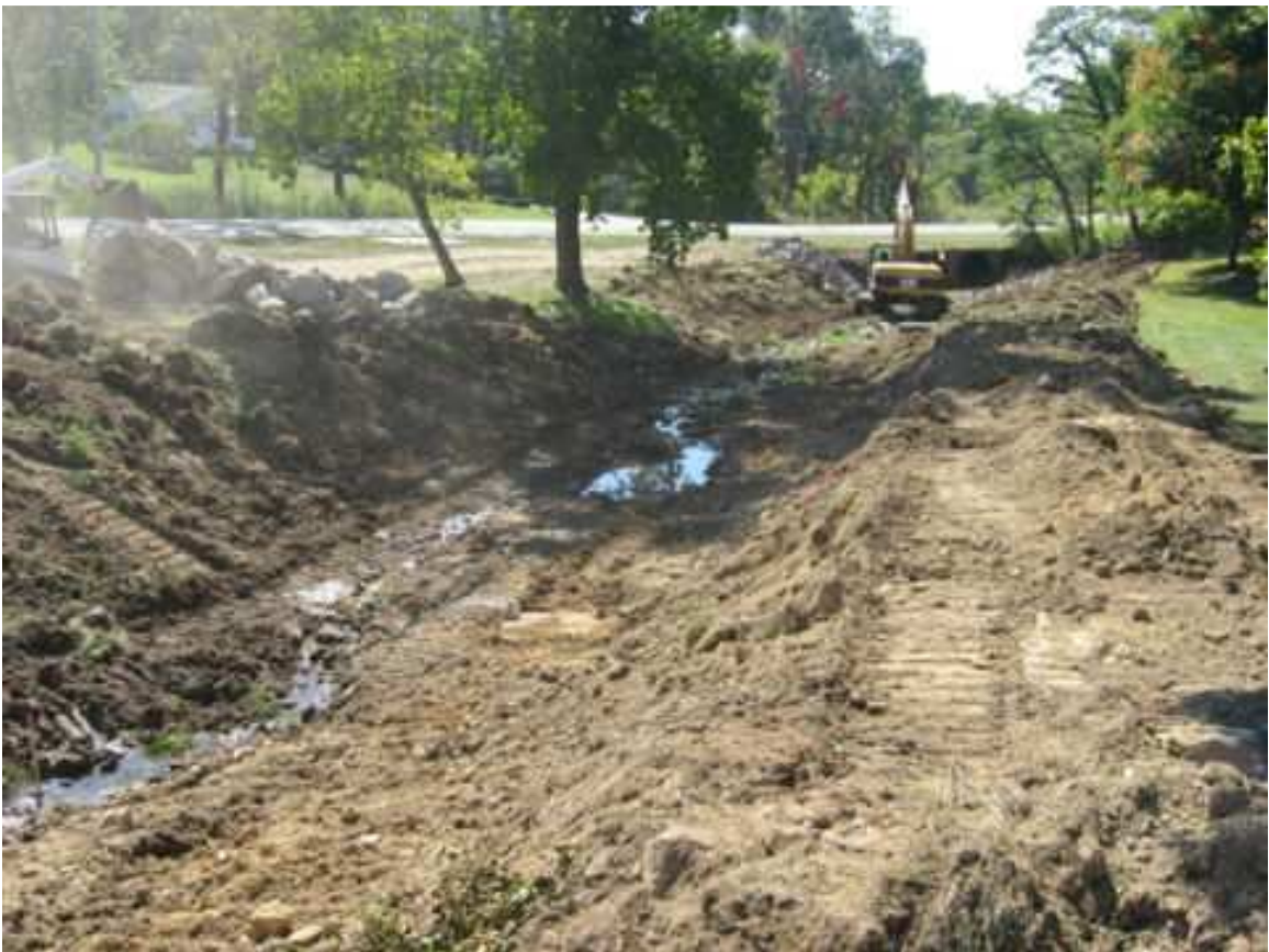
Figure 2.12 Widening of stream channel for Austintown Park restoration project (WPI 2008).
