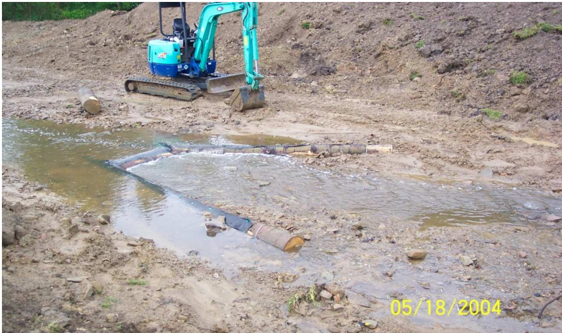
Figure 2.19 Finished log cross vane structure in Indian Run (WPI 2004).
