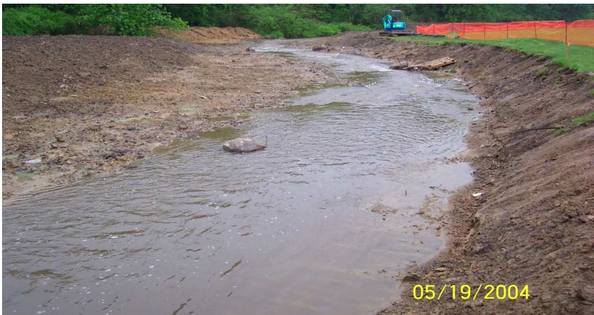
Figure 2.18 Widening of Indian Run stream channel (WPI 2004).
