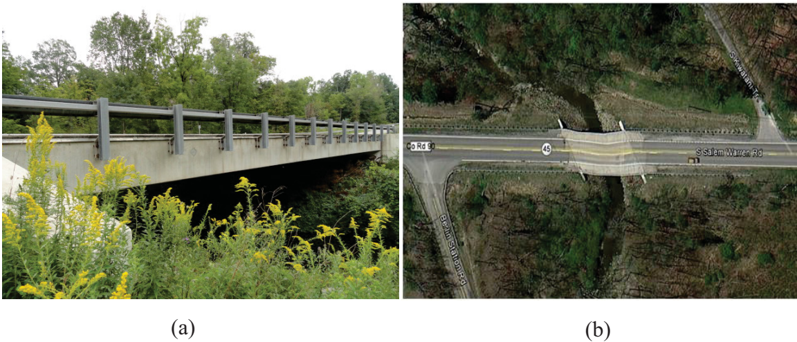
Figure 2.1: Mahoning Bridge: (a) side view, (b) top view (Google Map).
