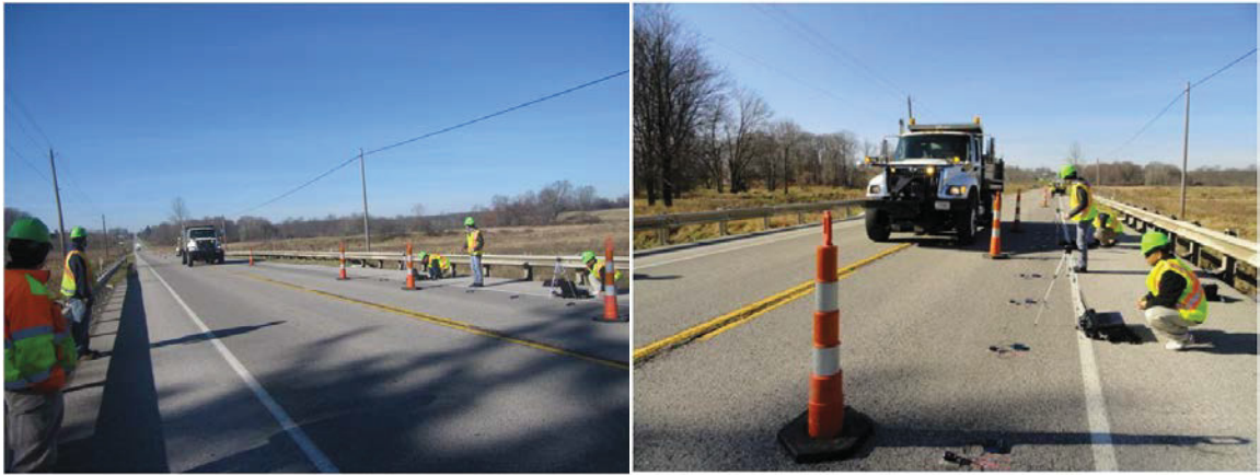
Figure 2.8: A test truck approaching to Ashtabula Bridge.
