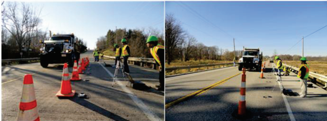
A: Data collection on MAH Bridge
