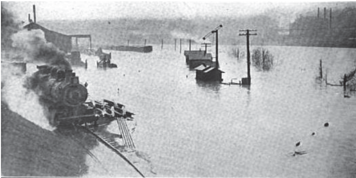
Figure 2-6: Completely submerged freight yard of the Pennsylvania Railroad Company's Youngstown facility following the 1913 Flood. This photo first appeared in Railway World , Vol. 57 in March, 1914. Despite the dangerously flooded tracks, a steam locomotive can be seen on the left side of the photograph.
