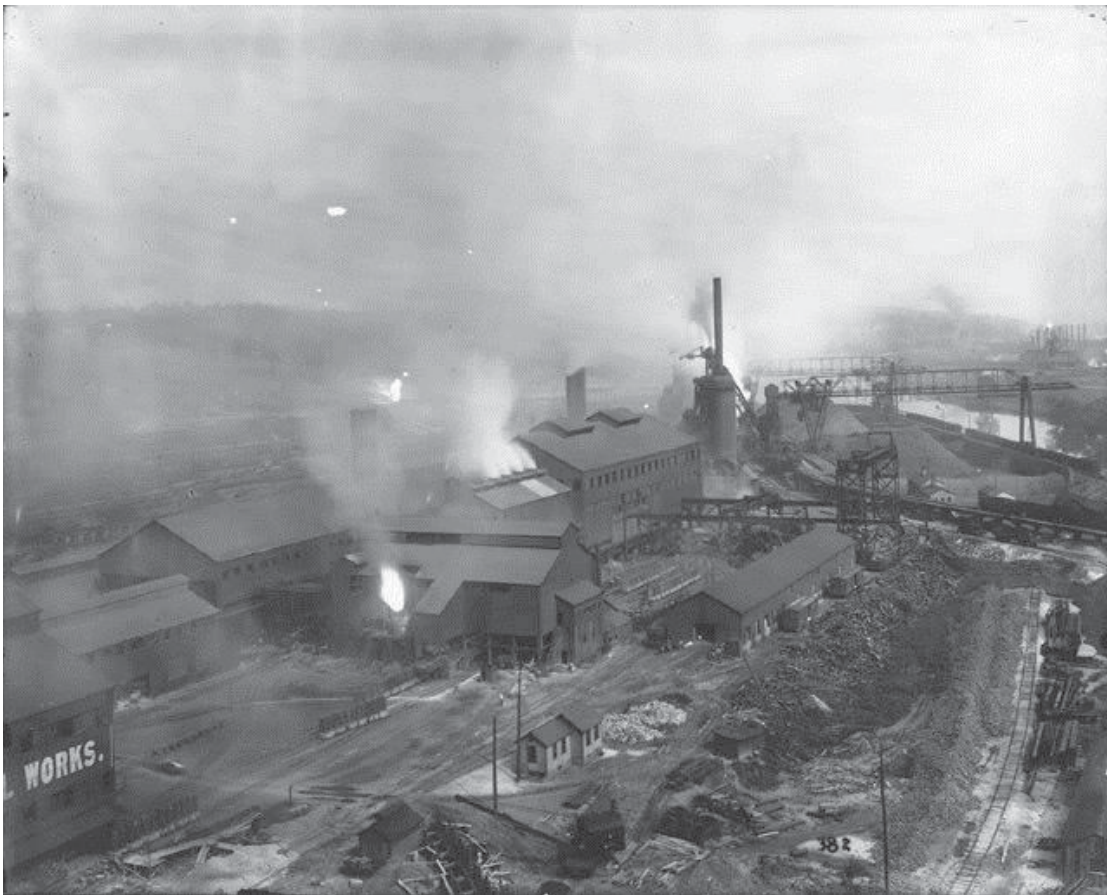
Figure 2-2: Youngstown Sheet & Tube's Campbell Works was an integrated mill capable of converting ore into liquid iron as well as converting pig iron into liquid steel. The casting process (transforming liquid steel into solid blocks) and blast furnaces on site required large amounts of water from the nearby Mahoning River. Circa late 1910s.
