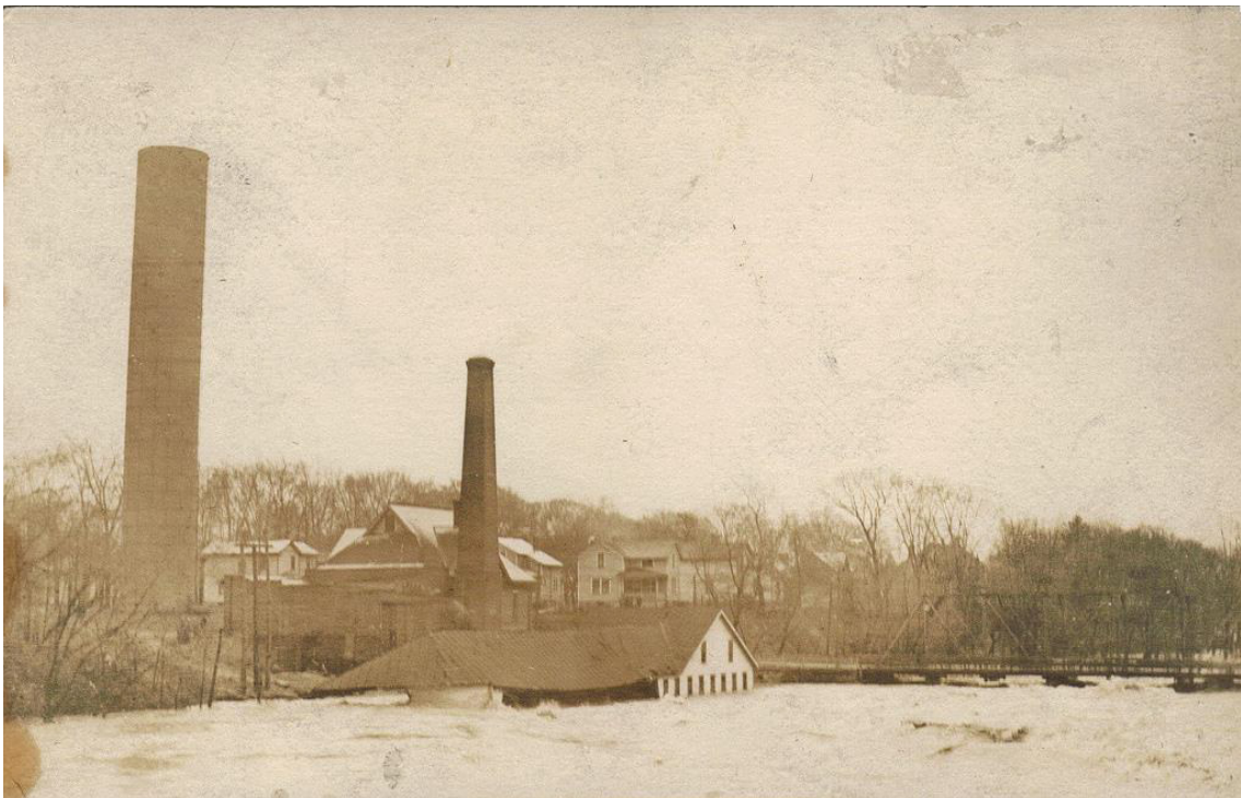
Figure 1-2: The water filtration plant located along the Mahoning River's edge at the intersection of Mahoning Ave. and Summit St. in Warren, OH was completely inundated when the floodwaters crested at more than ten feet above critical levels. Located approximately 20 miles NW of downtown Youngstown, the scene in Warren was typical of cities located near rivers in the Midwest.
