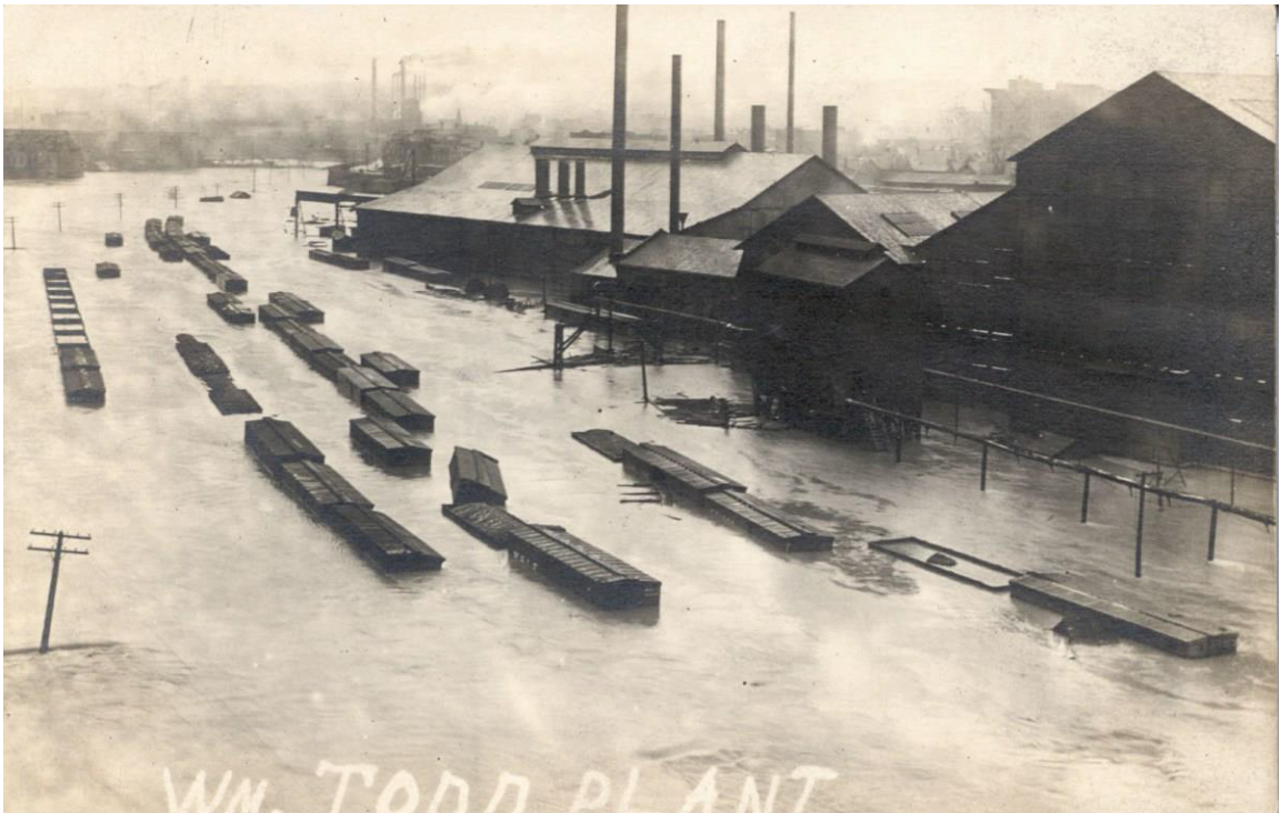
Figure 1-3: Situated just blocks from downtown Youngstown, the flood devastated the William Todd plant. After water breached the banks of the Mahoning River, it continued over the railroad tracks which serviced the integrated mill and eventually rose to levels which covered the floors of the mill and damaged machinery. Photo taken March 26 or 27, 1913.
