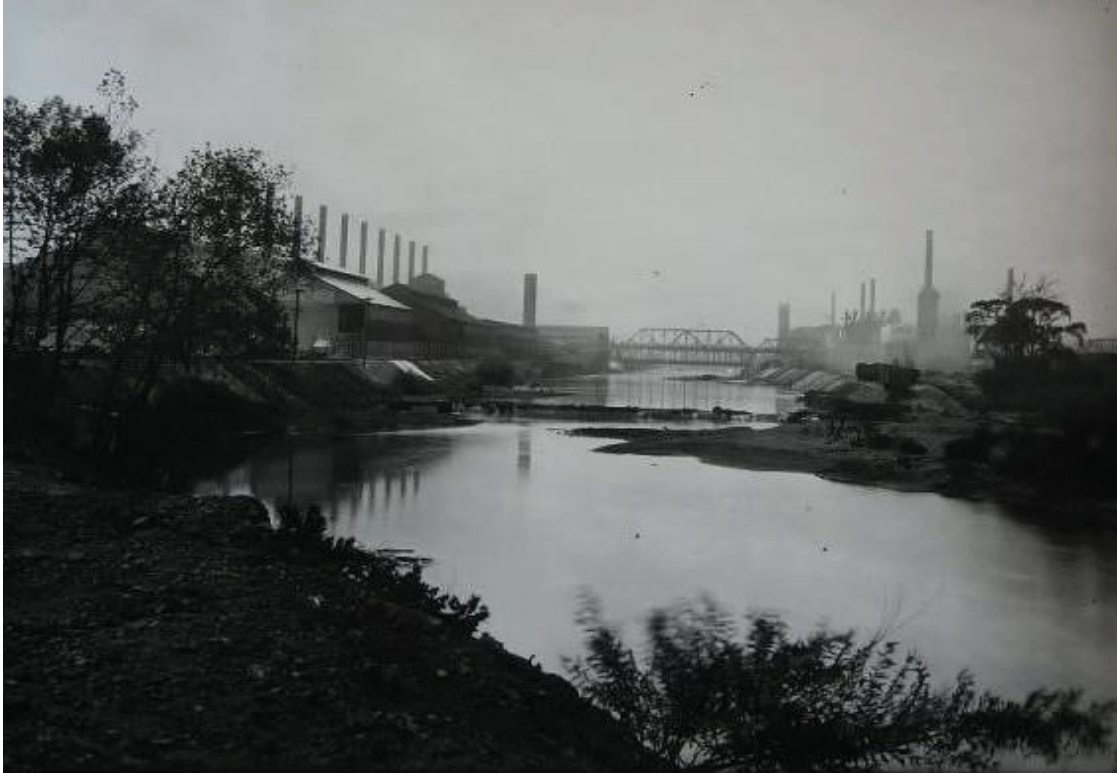
Figure 2-5: View of the Mahoning River during the dry season. Note the shallow water barely covering the riverbed at several points. Even along the banks the water level was low. Industrial water usage from mills such as Republic Steel's Haselton Works (seen here) placed heavy demands on the river due to its usage in cooling and steam production in blast furnaces. (Circa 1910).
