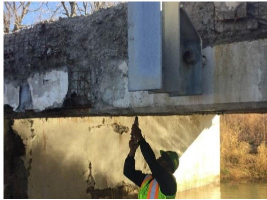
b) Schmidt hammer rebound test
