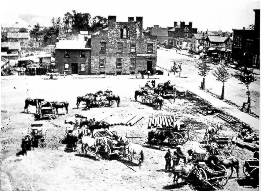
The north side of the Diamond is shown in 1872 at a time when they were preparing to lay water pipes. The view is down E. Federal St., with the Youngstown House where the People's Bank is today.
