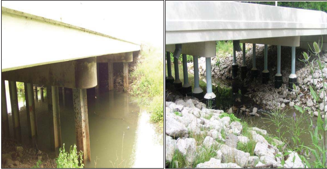
Figure 2-1: H-Pile- a) pier before encasement and b) pier after encasement
