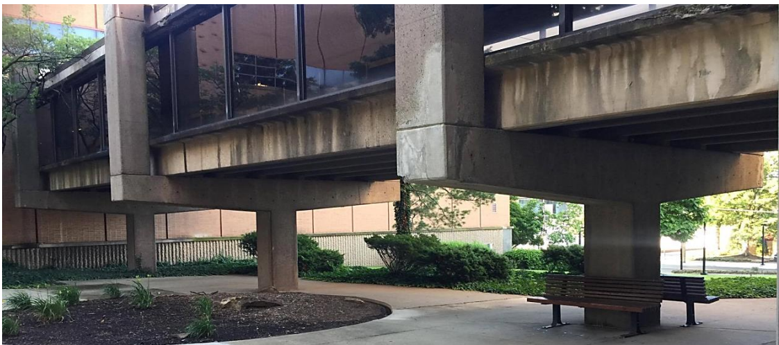
Figure 1-1: Pier caps supporting bridge between Moser and Cushwa Hall at YSU.
