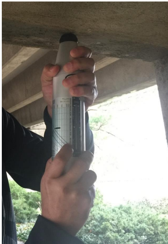
Figure 4-7: On-site Rebound hammer test.
