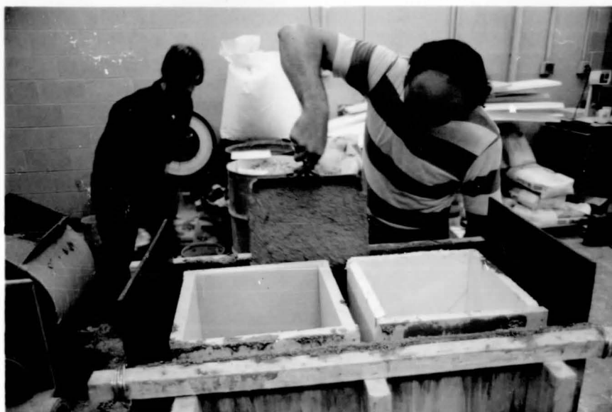
FIGURE 2.18 POURING LIGHTWEIGHT CONCRETE INTO MOLD FOR PROTOTYPE MODULE
