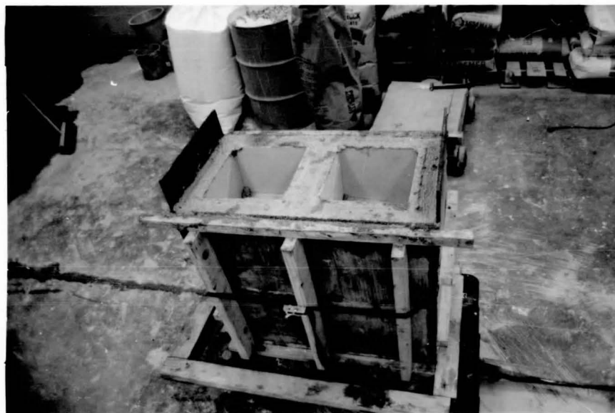
FIGURE 2.19 PROTOTYPE MODULE MOLD AFTER CONCRETE HAS BEEN POURED
