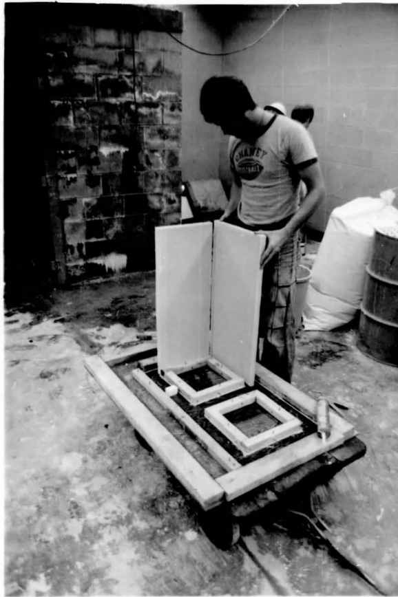
FIGURE 2.16 PLACING STYROFOAM SHEETS TO FORM RECTANGULAR VOIDS
