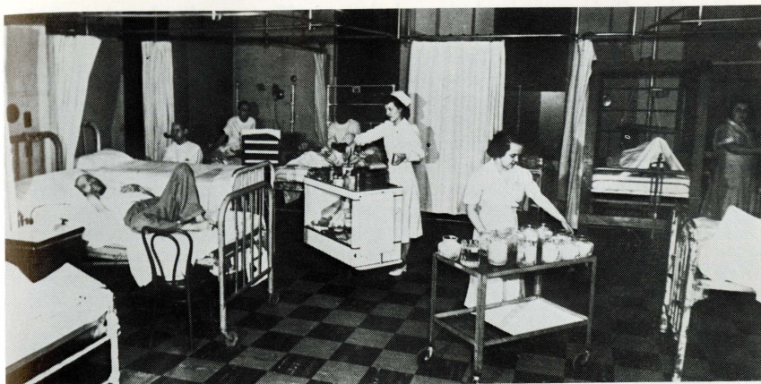
J Ward, South Unit (1912)
