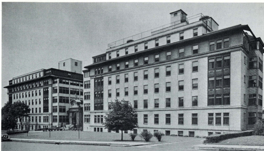
In 1929, the North and South Wing were joined by a lobby entrance.
