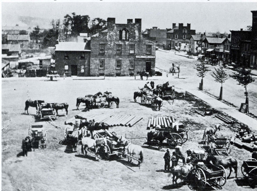
The north side of the Diamond is shown in 1872 at a time when they were preparing to lay water pipes. The view is down E. Federal St., with the Youngstown House where the People's Bank is today.
