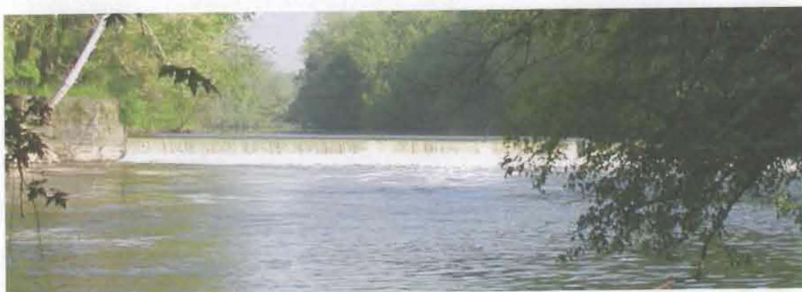
Liberty Street Dam, Girard OH
