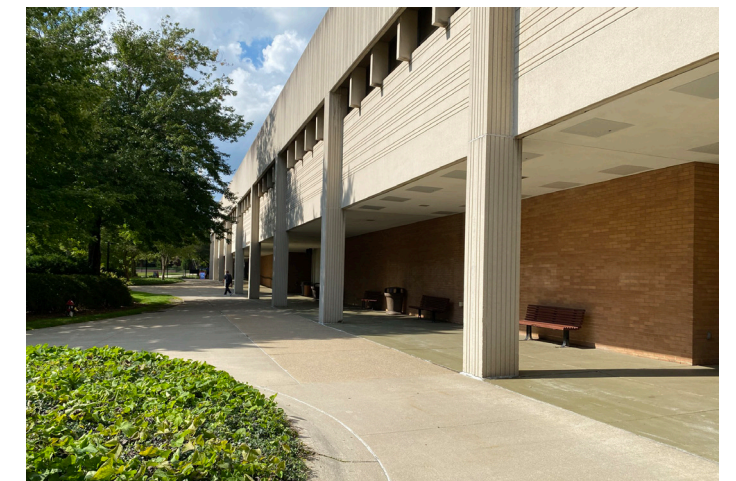
Current view of the Kilcawley Center from the main campus quad. The existing building lacks transparency from one side of the building to the other. The reimagined union on this site would include a "main street" through the building that would connect the north and south entrances.
