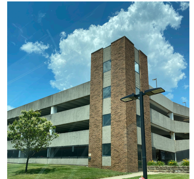
Current Parking Deck at 5th and Lincoln planned for demolition in the next couple of years
