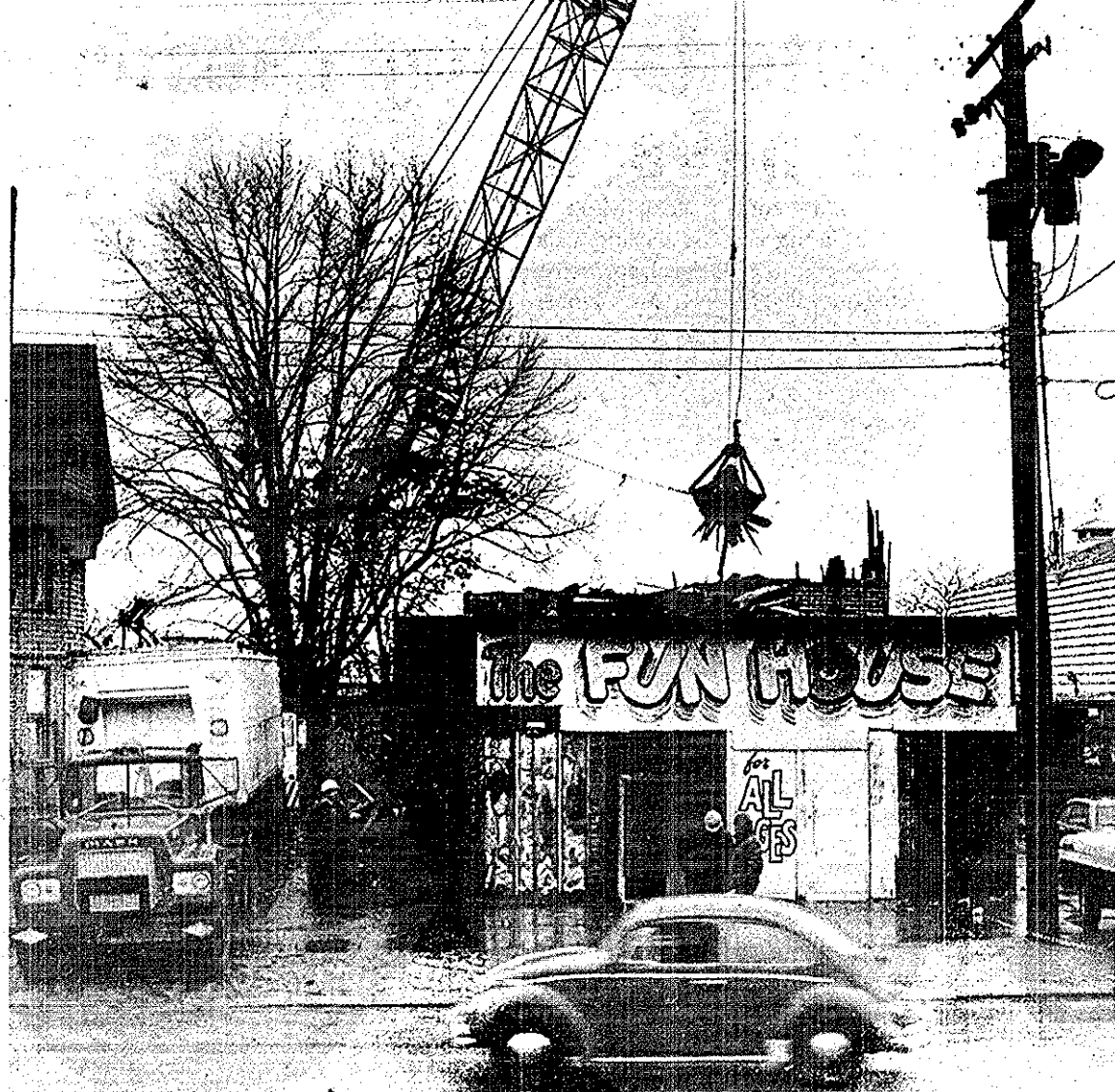
A NEW NIGHTSPOT —The Bavarian House recently purchased the building formerly known as the Funhouse which was gutted last year by fire. The middle of the structure has already been torn down, making it one long building without divisions inside. The new owners say it will take about four months for complete renovation of the future nightspot.
