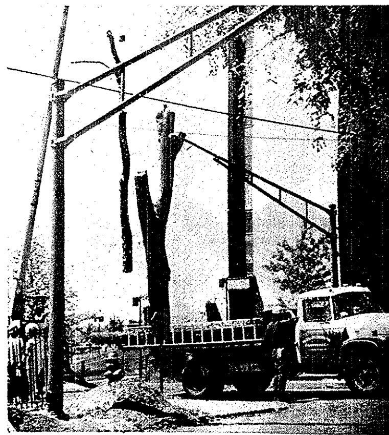
MORE TREE REMOVAL - The corner of Bryson and Spring Sts. was the scene of yet more tree felling on YSU's campus.
