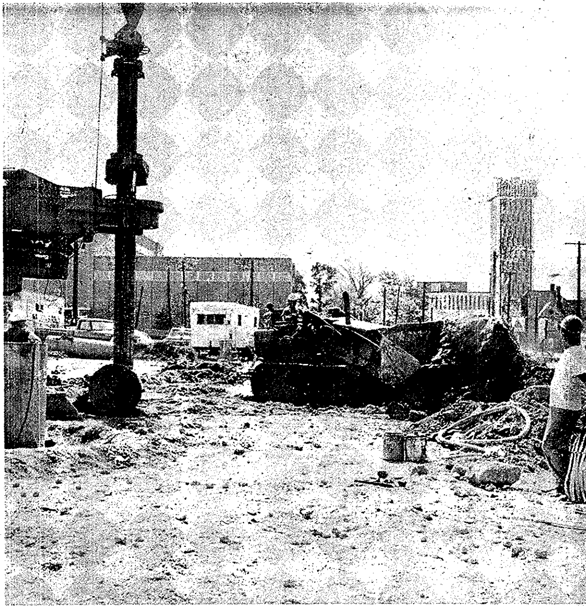
BULLDOZER FILLING — A Bulldozer, operated by Dan O'Connell, fills in dirt by construction site of new parking decks.
