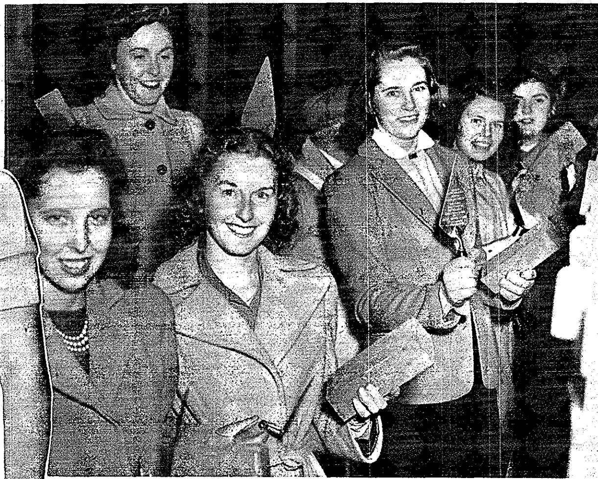
They Just Can't Wait — Co-eds at Colby College, Maine, tried to rush construction on their new gymnasium by helping lay bricks after the cornerstone exercises recently. Left to right are: Mary Weeks, Shirley Elice, Vivian Maxwell, Ann Westing, Nancy Grahn, and Mary Watson. Ann Westing wangled the silver cornerstone trowel for her work. Collegiate Digest Photo by Gray
