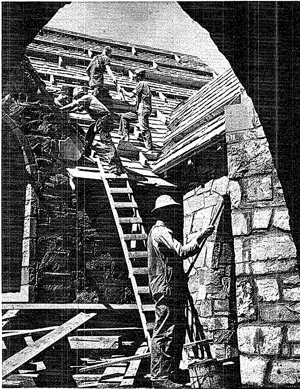
Male students are shown at work on another house for their school. They have also made all of the materials such as bricks, lumber, etc. The school is now an incorporated town.
