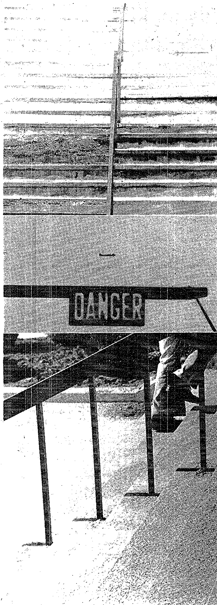
CRUMBLY CONCRETE CREATES CRACKS AND CREVICES - A combination of adverse weather conditions, salting, and possibly faulty mixing have created slowly deteriorating steps around the campus. Most noticeably affected are the Bookstore (left) and the new Maag Library (bottom).
