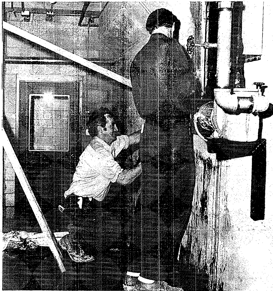
WHO PULLED THE PLUG? — Workmen brace window and apply extra caulking around the pane to prevent further leaking under the pool in the Beeghly Physical Education Building. The pool will be opened Monday for class.
