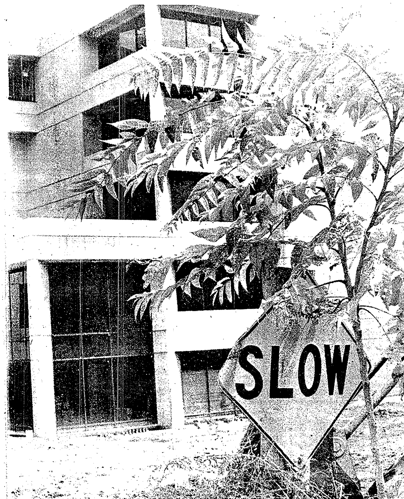
Front cover photo: Whoever put up the street sign in such an unlikely place definitely knows the score as far as construction of the Maag Library goes. The new library (background) has been under construction for almost four years now, and nobody knows for sure when it will be finished.
