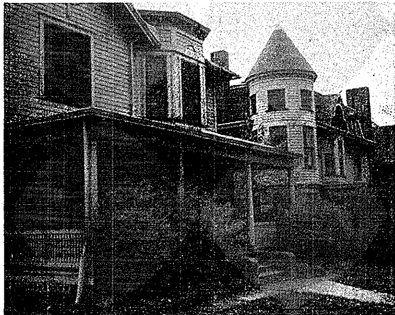
This group of houses will be torn down to make way for the new Science Building. A date has not been set to begin construction.
