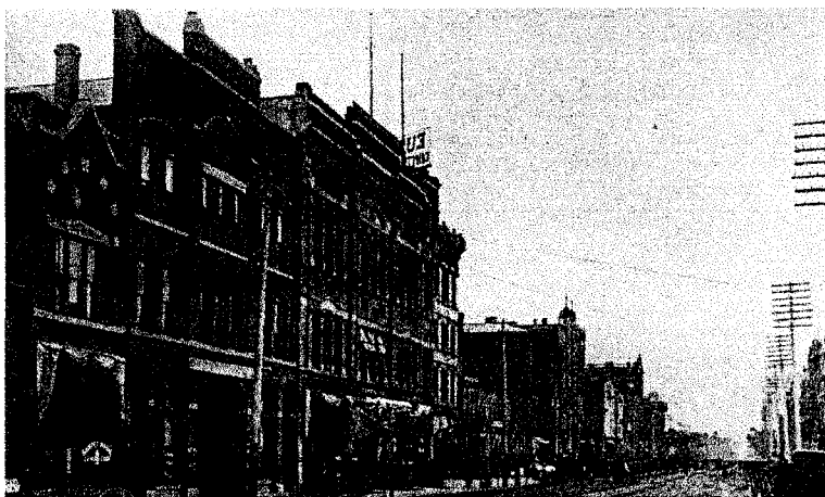
fig.11 West Federal Street Looking east
