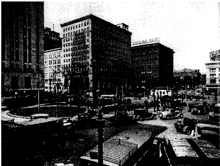
fig.29 Central Square c.1930 Looking north
