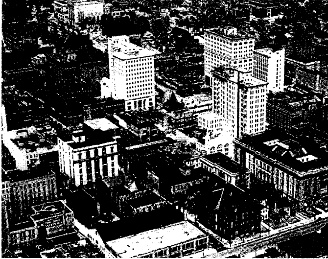
fig.30 Central Square c.1930 Looking north
