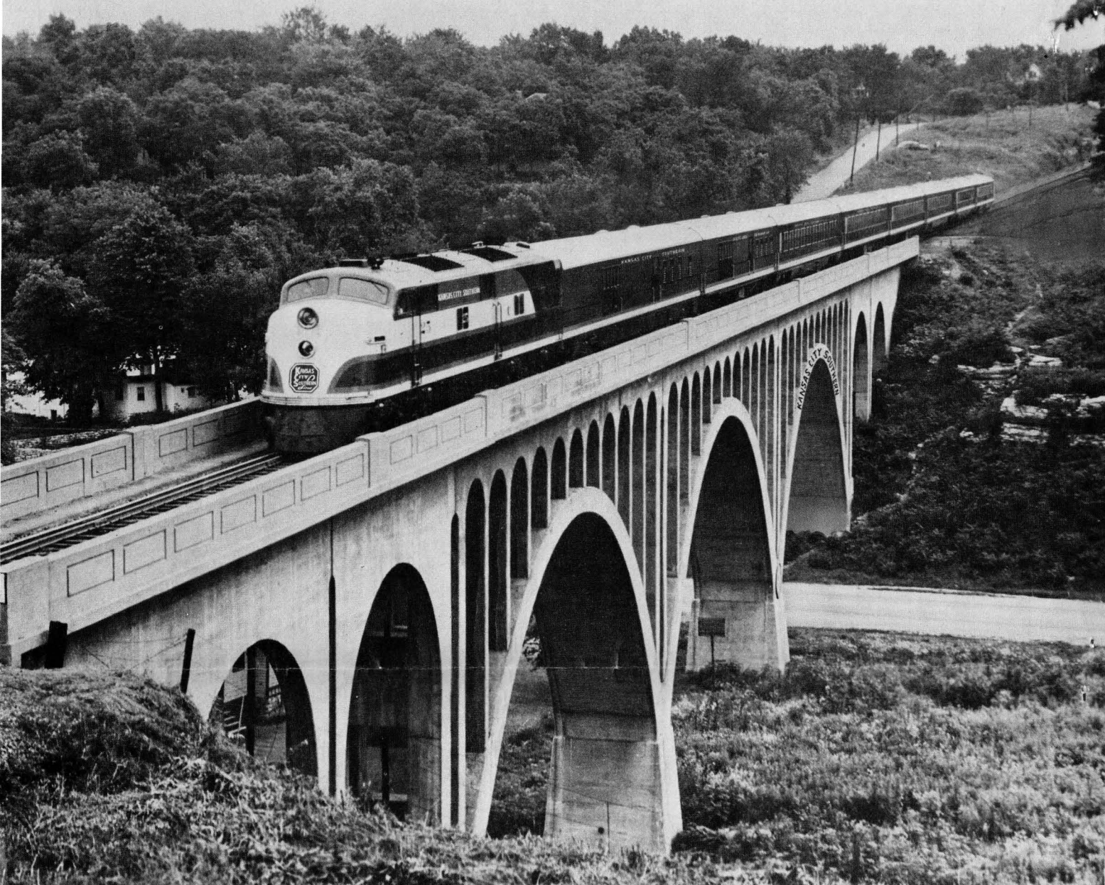
Southern Belle of Kansas City Southern crossing one of the large and graceful viaducts of the railway near Kansas City, Mo., in mid-1950s.
