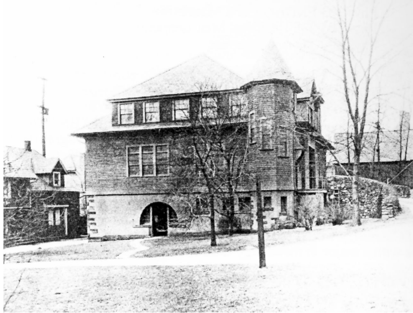
Applied Science Building
