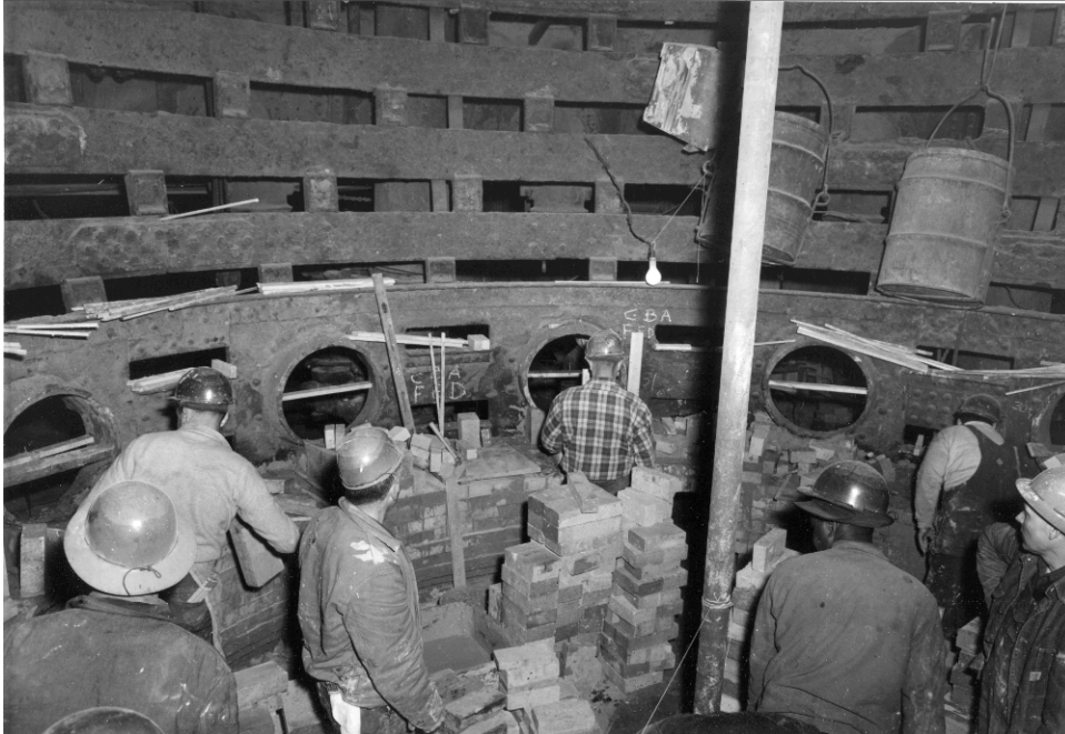
Figure 4-10: In January 1955, Sheet & Tube invested one final relining of the Hubbard furnace. This rare look inside the Hubbard furnace shows Sheet & Tube personnel relining the stack at the level of the tuyeres just below the bustle pipe in the furnace's hearth. The bricks used in the reline averaged seven to fifty pounds. The 1955 reline was Sheet & Tube's last major investment at its Hubbard stack and operations only continued for another five years.
