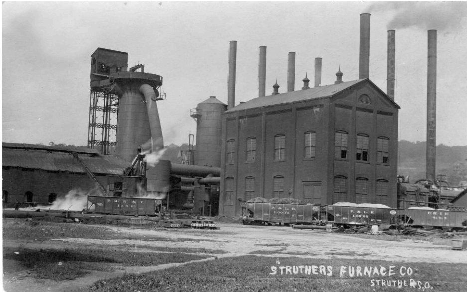
Figure 1-2: Prior to its rebuild in 1909, the Anna furnace remained a relatively old stack that retained an 1890s build. Shown from l. to r. are the furnace's cast house, elevator hoist and Anna furnace, firebrick hot stoves (behind the blowing engine house), blowing engine house, and boilers. The blowing engine house, constructed in the early 1890s, housed one Weimar and two small Cuyahoga high-pressure steam-blowing engines.
