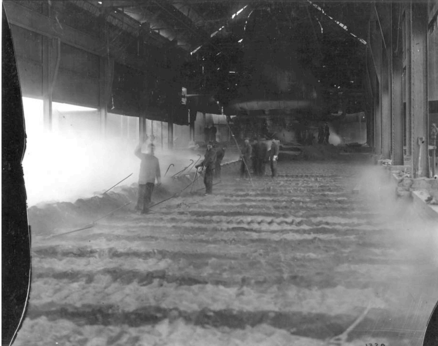
Figure 2-4: The image above shows a view inside the cast house of Lowellville’s Mary furnace c. 1908-10. The furnace is shown in the background with employees using trowels to direct the flow of the iron on the sand bed-casting floor. Workers directed the iron into molds, which cooled and formed hardened pig iron. Men wielding sledgehammers broke the iron and loaded it onto railroad cars for shipment. By 1910, the Hubbard furnaces and Mary furnace were the last in the Mahoning Valley to exclusively cast pig iron with this outdated and laborious method.
