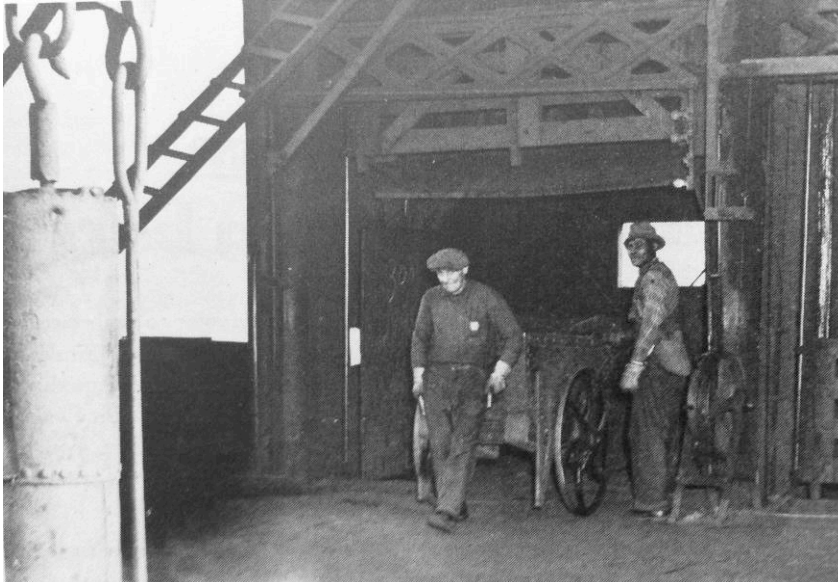
Figure 2-11: A top filler removes a barrow full of coke from the unloading platform at the furnace's top in the late 1940s. Although gas-operated forklifts removed much of the labor for the bottom fillers, the top fillers still had to handle 700-1,000 pound barrows of both iron ore and coke and dump the materials evenly on the furnace's hopper.
