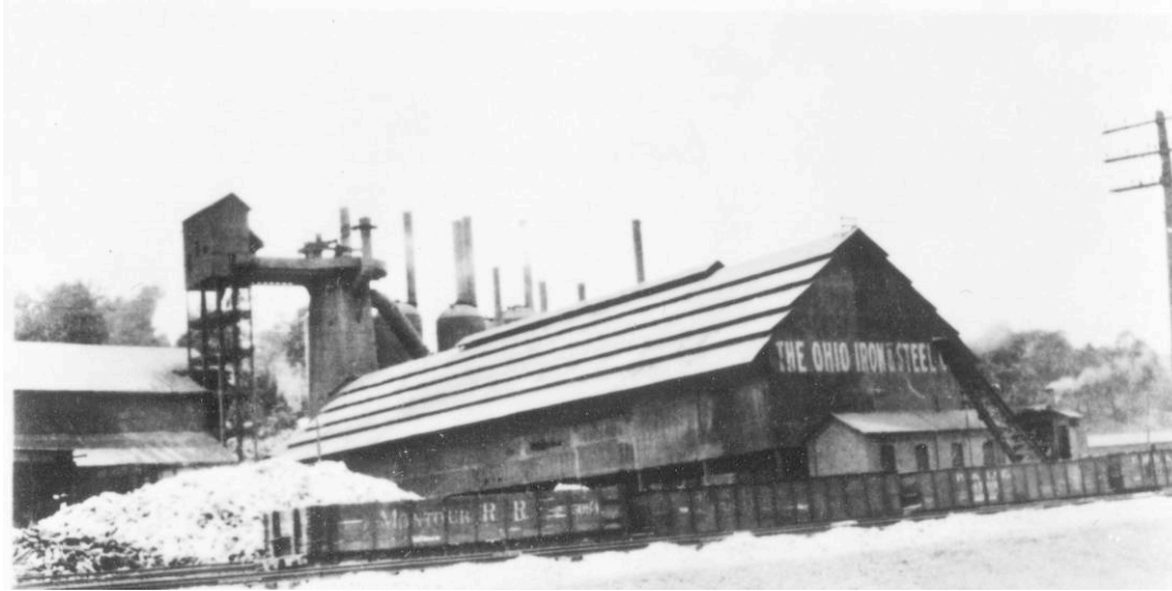
Figure 2-3: The Ohio Iron and Steel Company's Mary furnace is pictured here around the turn of the twentieth century. Shown from left to right is the furnace stock house, elevator hoist, furnace and its long cast house with hot stoves in the background. The extended cast house accommodated the enlarged capacity of the furnace after its enlargement in 1898.
