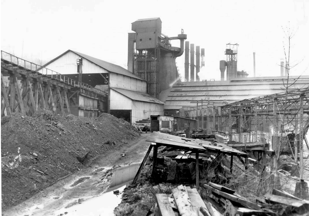
Figure 2-14: This c. 1960-61 photo shows the Mary furnace shortly before its abandonment. At left are the furnace’s stock house, wooden ore trestles and iron ore pockets. Unlike most pioneer and merchant furnaces in the valley, Mary furnace still retained old wooden trestles, a method that other furnaces abandoned by the 1920s. The furnace also still utilized wooden ore pockets, a system of iron ore distribution that allowed workers to pull a lever, thereby opening a door and allowing iron ore to fall into their barrows via gravity, the same method used at Hubbard furnace from 1900-1920.
