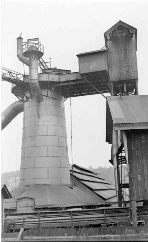
Figure 2-1: Built in 1845, Lowellville's Mary furnace was the first in the United States constructed to intentionally utilize raw coal as fuel. By the mid-twentieth century, it was the oldest active furnace in both the Mahoning Valley and the world, and retained a unique aspect of old blast furnace practice for its entire lifetime: hand-fed charging rather than automatic skip charging. This 1932 image shows the furnace, its elevator hoist and old wooden stock house at right.
