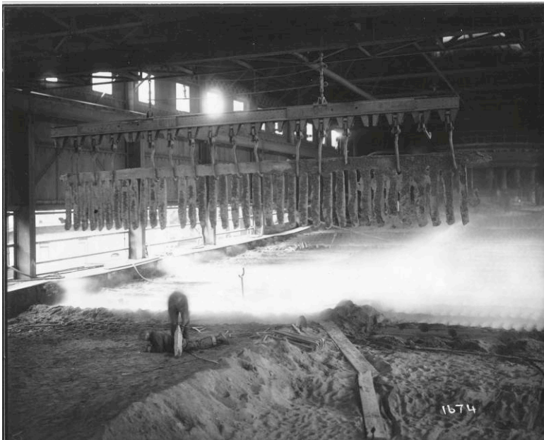
Figure 3-6: Inside the cast house, iron was still cast in sand molds on the furnace floor. The image above shows a comb of hardened pig iron being carried to the pig breaker, where they were mechanically broken, rather than the old method of laborers manually breaking the iron with sledgehammers.
