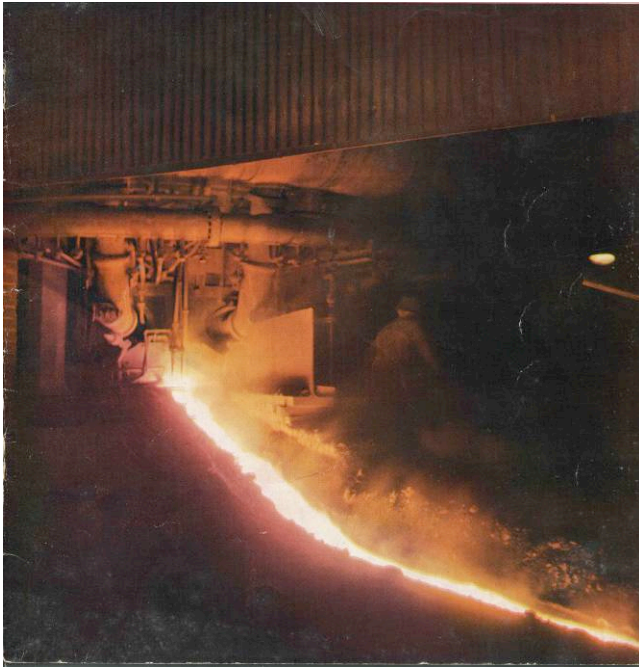
Figure 2-6: After Sharon Steel Hoop purchased the Mary furnace in 1918, all iron was cast through runners and into ladles for transport to the company's nearby open-hearth steel plant. The company used the casting machine primarily on Sundays when the steel works closed. This photo shows molten slag running through troughs on its way to the slag pit at Mary furnace in the early to mid 1940s. The slag, or cinder notch, was located slightly above the iron notch because molten slag floated on top of the iron within the hearth.
