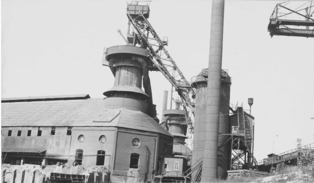
Figure 4-7: This 1932 photo shows the Hubbard furnaces idled due to the depression. In Lowellville and Struthers, both the Mary and Anna furnaces were also idled until conditions improved enough for the aged furnaces to be profitable. The Hubbard No. 2 furnace (foreground) was dismantled in September 1937.
