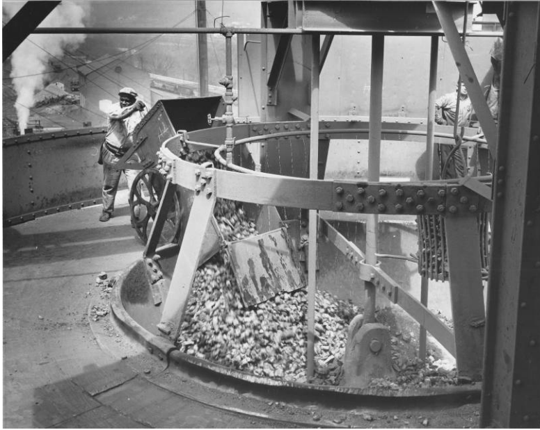
Figure 2-12: This 1957 photograph shows a top filler dumping coke onto the Mary furnace's hopper, which was then lowered into the stack. The rigging system on the furnace's top is shown here with a water spray system to moisten the burden and steel bars that prevented the barrow from accidentally falling on the bell and hopper. The furnace's ladle house is shown in the background.
