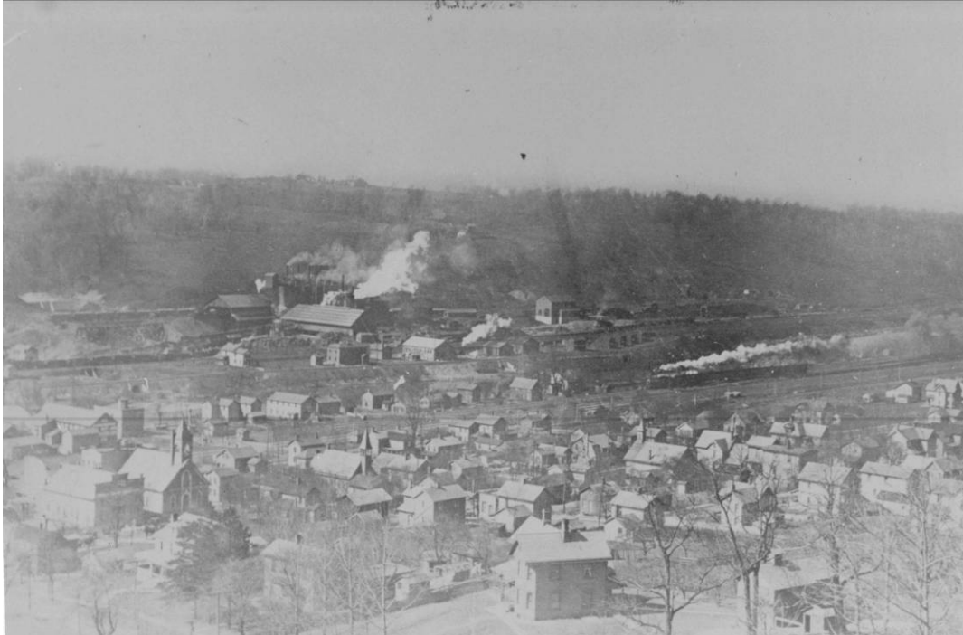
Figure 2-2: By 1900, the small village of Lowellville presented little heavy industry with the exception of the blast furnace. This c. 1912 view from Bedford Hill shows the Mary furnace in the distance, then owned by the Ohio Iron and Steel Co., which formed in 1880. Although the company's name included the word "steel," it only produced pig iron from the Mary furnace to sell to foundries and steel mills, largely located in Pennsylvania and New York.
