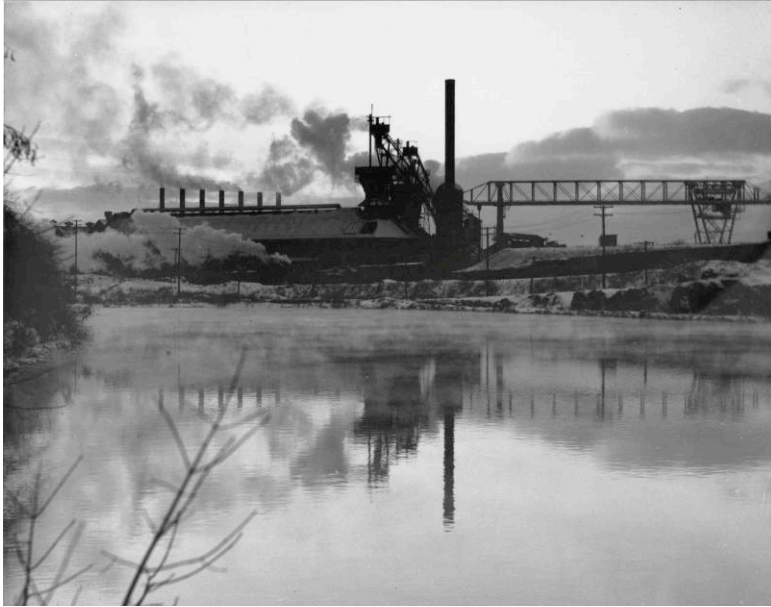
Figure 4-6: A c. 1930 view looking west along the Yankee Run reservoir of the two Hubbard furnaces and the new 10-ton Heyl & Patterson ore bridge to the right. The new Hubbard plant of the Valley Mould and Iron Co. is located to the right of the photographer. The new ore bridge and iron ore distribution eliminated much of the small labor positions at the furnace.
