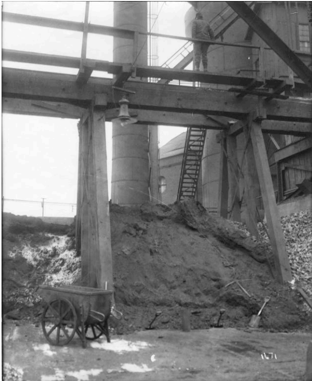
Figure 3-8: Raw material handling still remained fairly antiquated despite the modernizations to the furnace in 1910. This image shows iron ore piled underneath the 20-foot elevated wooden railroad trestles. Bottom fillers still had the laborious task of loading ore barrows with 500-700 pounds of iron ore and dumping them into the skip buckets.
