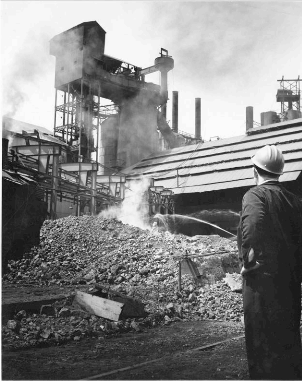
Figure 2-13: Despite being the oldest blast furnace in the United States and one of two remaining hand-fed furnaces in the world, Mary still operated and produced iron for the Sharon Steel Corporation's Lowellville Works throughout the 1950s. Shown in the midground of this 1957 photo are water sprays cooling and granulating slag as the elevator hoist lifts barrows to the top of the stack. Dave Rearick, who replaced long-time Mary furnace superintendent John Stewart in 1955, stands in the foreground.
