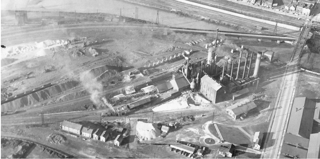
Figure 1-8: This late 1940s or early 1950s aerial view of the Anna furnace shows the plant's rather atypical layout along Bridge Street. The furnace's stockyard contained three trestles, one wooden (demolished in the photo) and two concrete. The plant did not utilize an ore bridge, but rather steam-powered cranes for raw material distribution, but it did contain stock bins similar to that of a modern furnace. Shown in the center of the photo is the furnace's Heyl & Patterson single strand pig casting machine.
