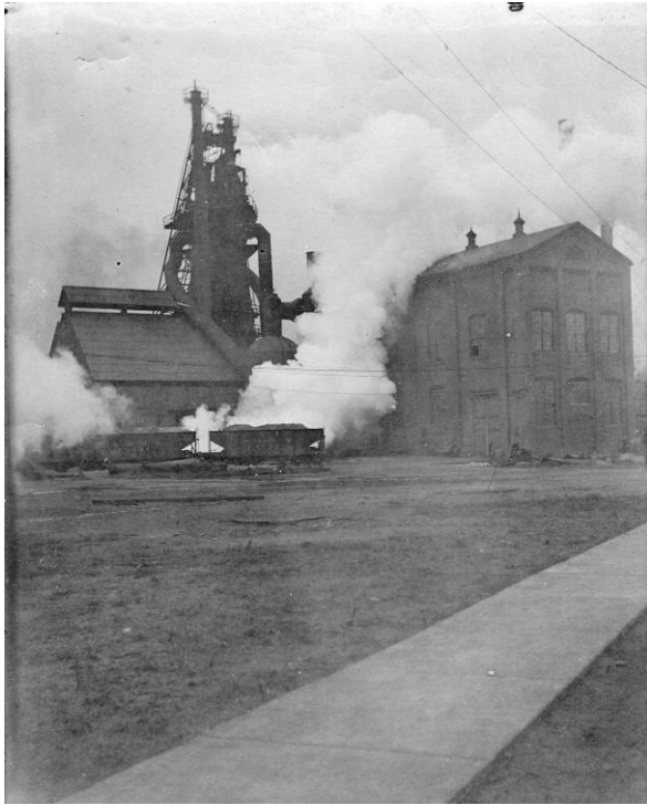
Figure 1-6: This photo shows the Anna furnace in operation in 1914. The coming of the First World War shot pig iron prices up to a price not seen since the Civil War in the Mahoning Valley. The Struthers Furnace Company maintained full operation through the war years and produced both foundry and basic pig iron for open-hearth steel works.
