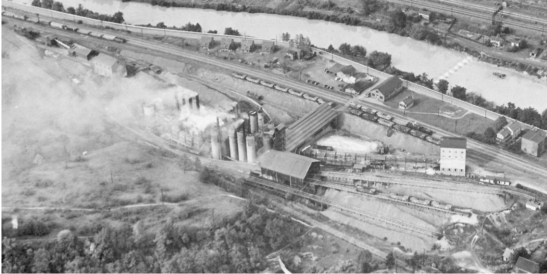
Figure 2-7: An aerial view of Sharon Steel’s Mary furnace in the 1940s shows the configuration of the small blast furnace plant. The Mary furnace still maintained blast furnace operations similar to those used in the 1890s. The furnace’s ore trestles and slag house are on the right side of the image, and the ladle house and pig casting machine are seen at the top left.
