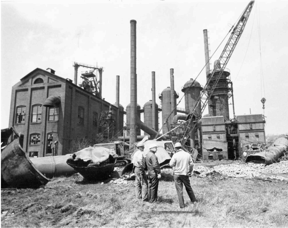
Figure 1-10: J. D. Fowler officials stand amongst the remains of the Anna furnace's boiler plant. The constant neglect and dilapidation over a period of thirteen years left shattered windows about the blowing engine house and plants sprouting around the furnace grounds. The dismantling of the Anna furnace left only the Hubbard stack as the last extant pioneer blast furnace in the Mahoning Valley.
