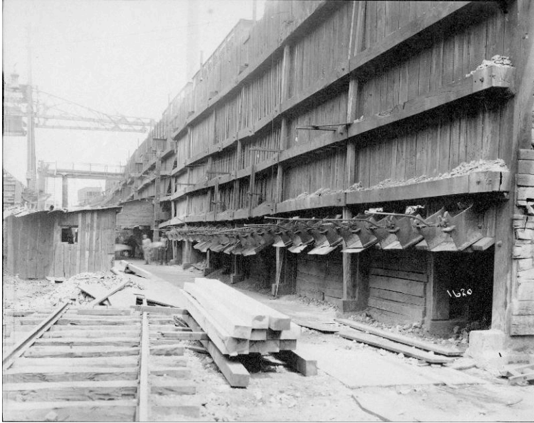
Figure 4-2: Prior to the installation of modernized stock bins in 1919, these make-shift, wooden-clad coke bins necessitated bottom fillers to pull a lever, which allowed coke to drop from the chutes via gravity into coke barrows. The barrows were then wheeled into the overhang seen at center left, where they were dumped into the skip buckets.
