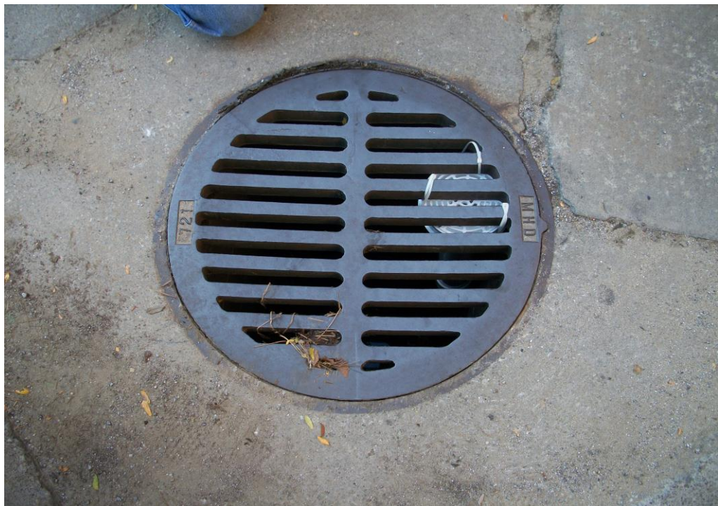
Figure 3.6: Storm Water Sampler Attached to Basin C-31.
