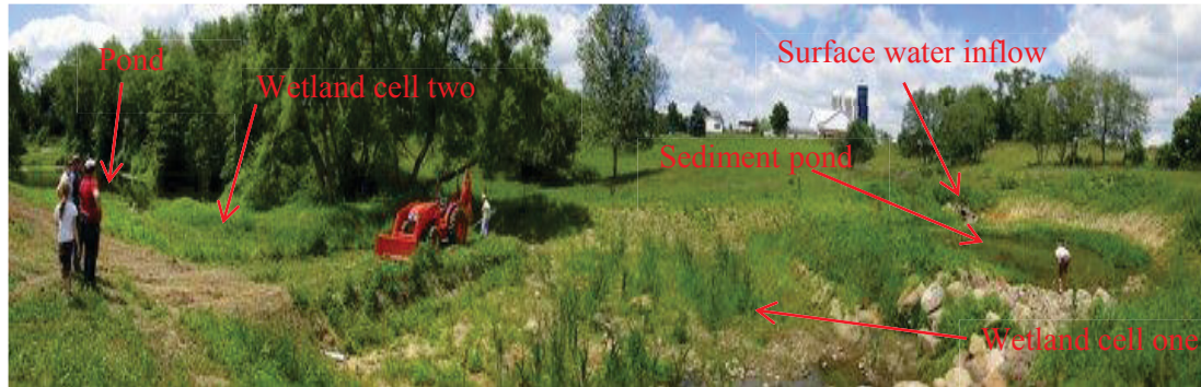
Figure 3.2: Constructed Wetland Showing Each Component
