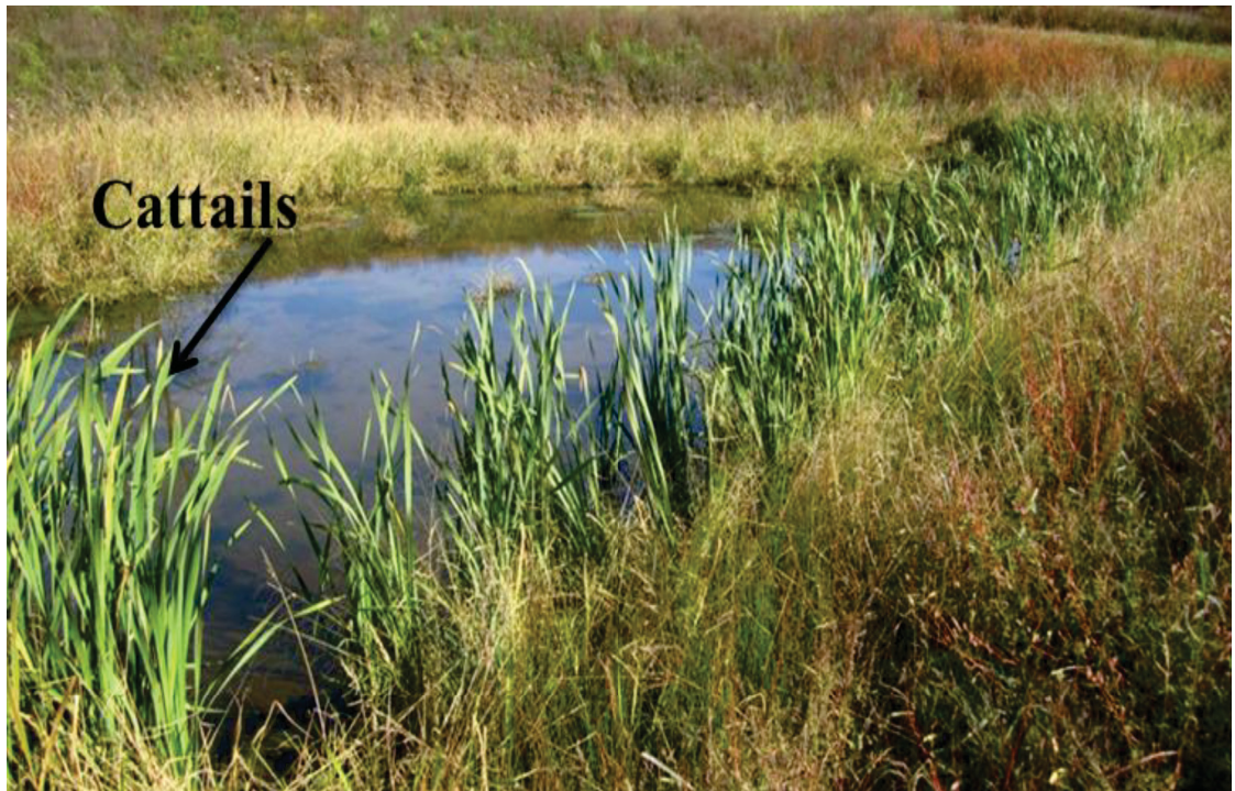
Figure 5.1: Sediment Pond with Cattail Growth
