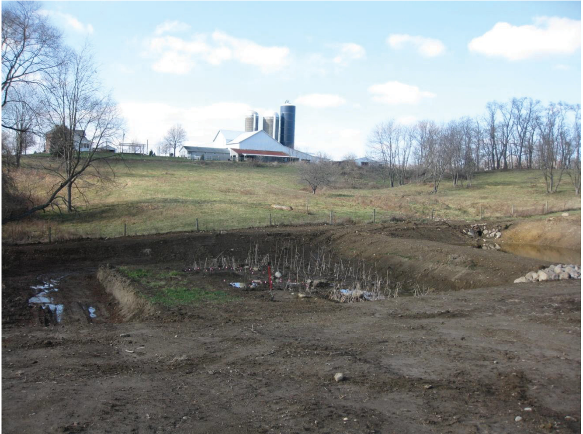
Figure 3.3 Settling pond (on right) and the constructed wetland cells.
