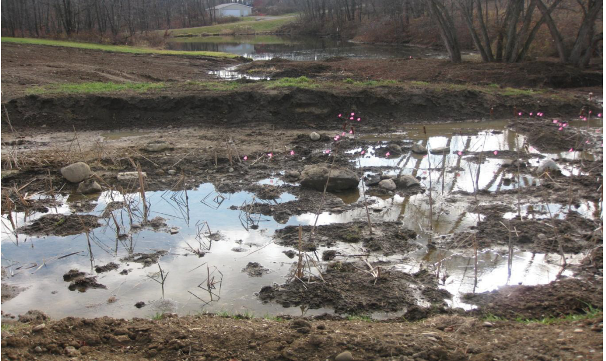
Figure A.5 Wetland Cell #1 after Construction
