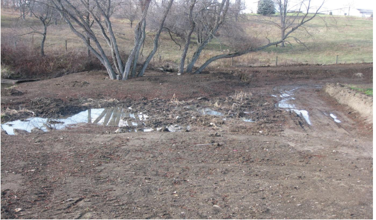
Figure A.9 Wetland Cell #2 after Construction
