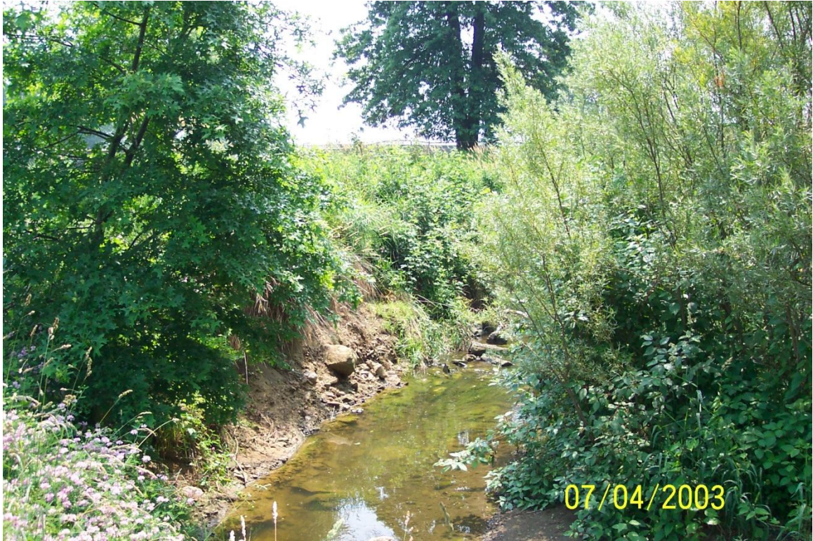
Figure 2-11. Right bank erosion in Indian Run (WPI, 2010).
