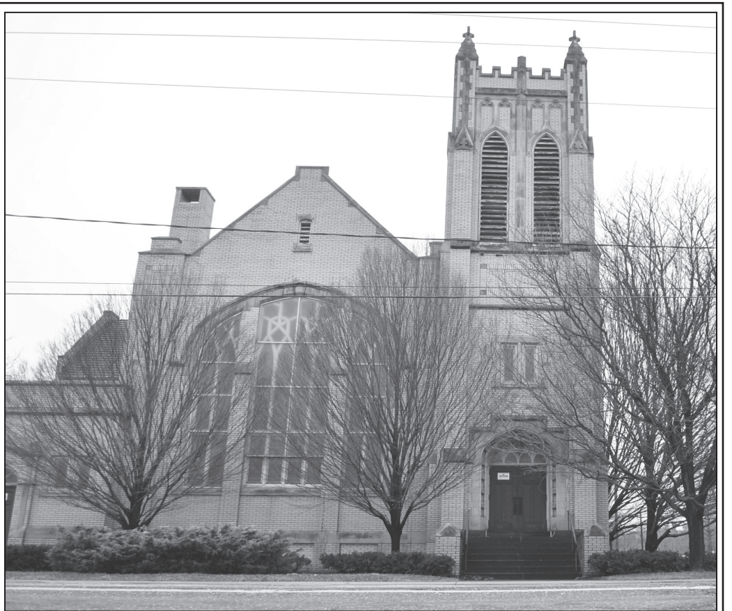
Dormant, Pilgrim Collegiate Church sits adjacent to Jones Hall. On Tuesday, the board of trustees decided to demolish the church, which YSU acquired in 2008. "We understand the emotions involved in decisions to demolish a building on campus; those emotions are particularly difficult when the building is a church," Gene Grilli, vice president for finance and administration, wrote in a memo. Grilli explained how various uses for the building were explored, yet all required excessive renovation costs which were unjustifiable. No official date is set for the demolition. Photo by Jordan D. Uhl/The Jambar.
