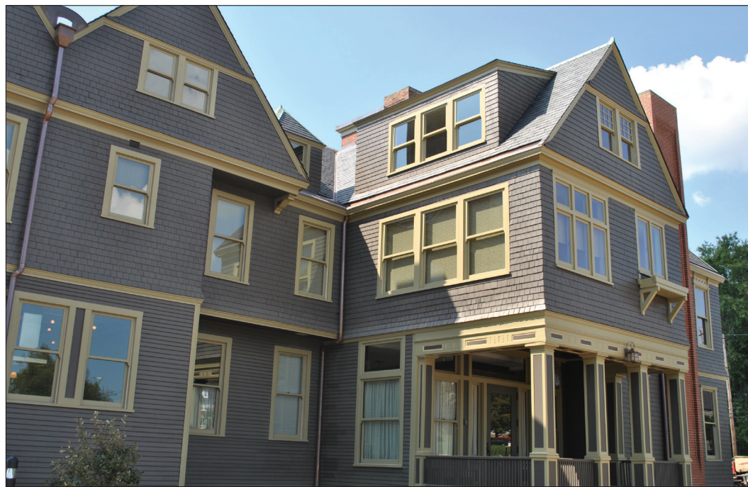
The YSU Board of Trustees took a tour through the newly remodeled Porter and Mary Pollock House on Thursday. The project cost $4.47 million. Photo by Kacy Standohar/The Jambar.
