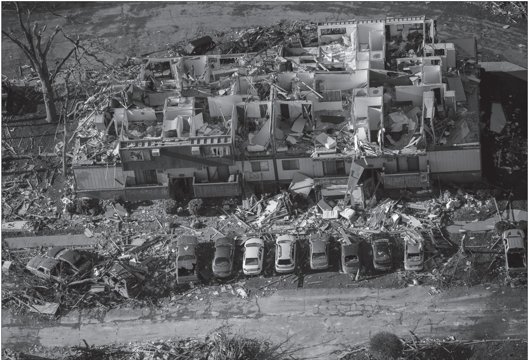
A multi-unit building and cars destroyed by the tornado in Washington, Ill., near Peoria is seen on Monday, Nov. 18, 2013. Zbigniew Bzdak/Chicago Tribune/MCT.
