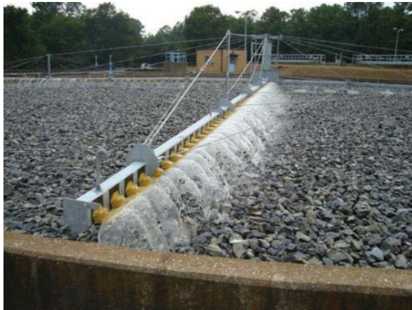
Figure 2.4: Typical distributors with rotary arms, used to apply wastewater to trickling filter packing (Kusters Water, 2014)
