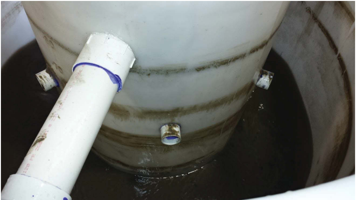
Figure C.10: IMET Process tank 4, side view of inner tank
