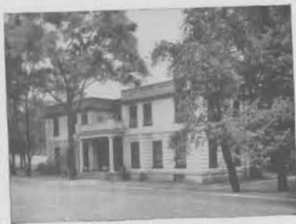
"Graybloe Hall" Service Building
