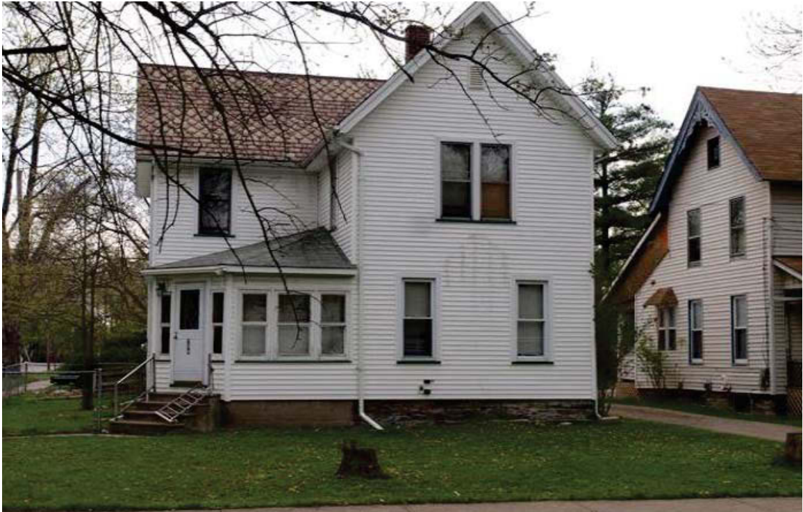
Figure 3 Photograph of the site showing the abandoned house prior to demolition.
