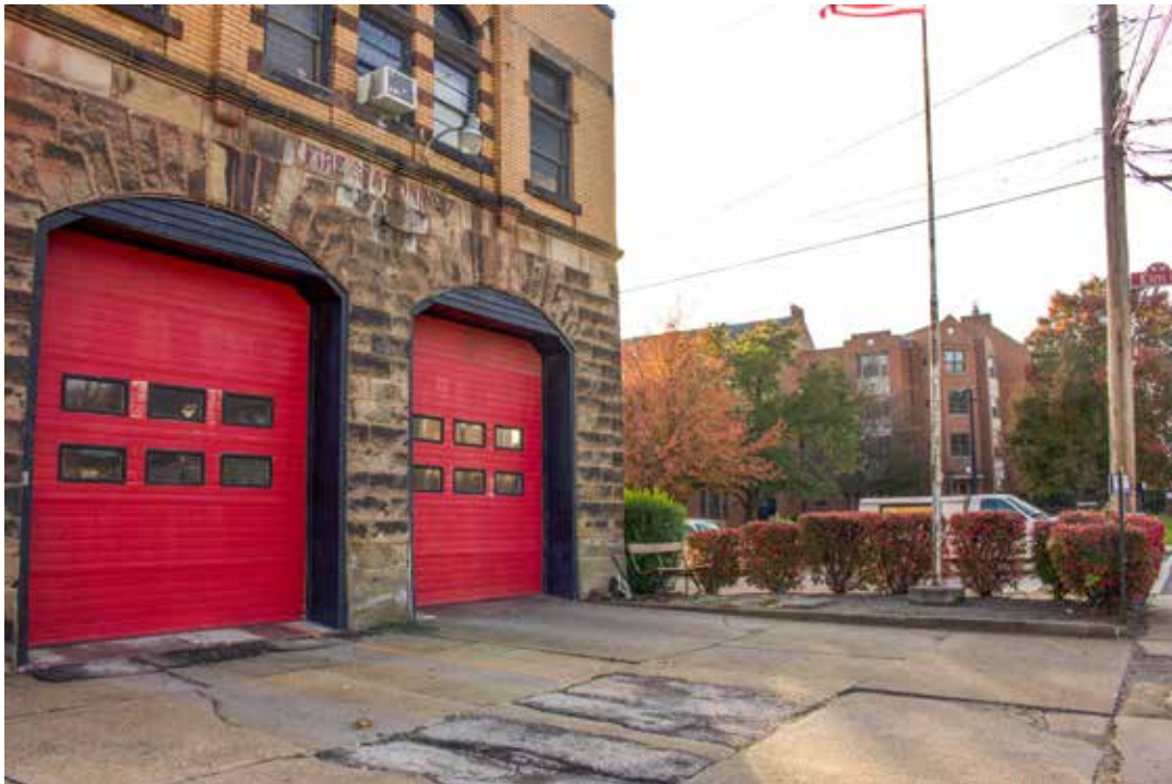
Youngstown's Fire Station 7 has been serving the Youngstown area for 116 years. Photo by Abigail Cloutier/The Jambar
