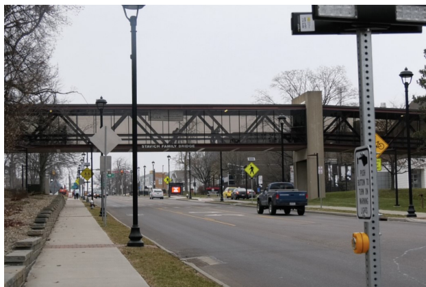
The roof will be replaced at Stavich Family Bridge, which connects the Wick Avenue parking deck to Meshel Hall and the rest of campus, over the summer. Photo by Jordan Boitnott/Jambar Contributor
