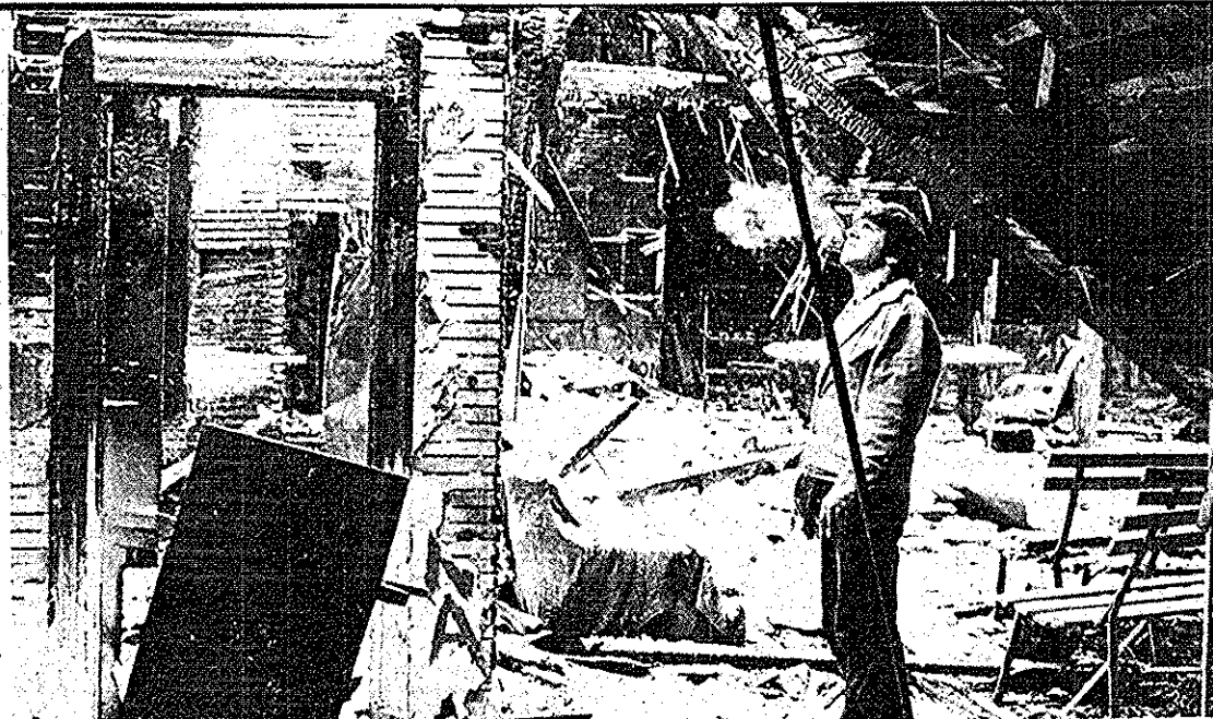
EXTENSIVE DAMAGE.— A Sigma Alpha Epsilon fraternity member surveys fire damage to a room on the second floor of the fraternity house on Pennsylvania Avenue. (Photo by Bill Oberman).
